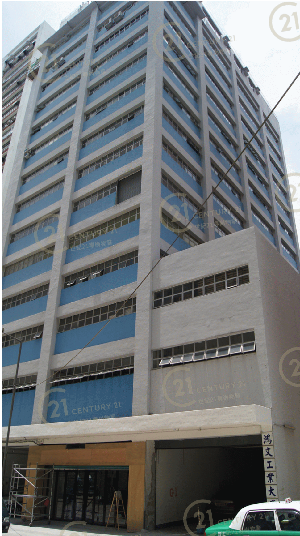
鴻文工業大廈 Chaos Industrial Building
