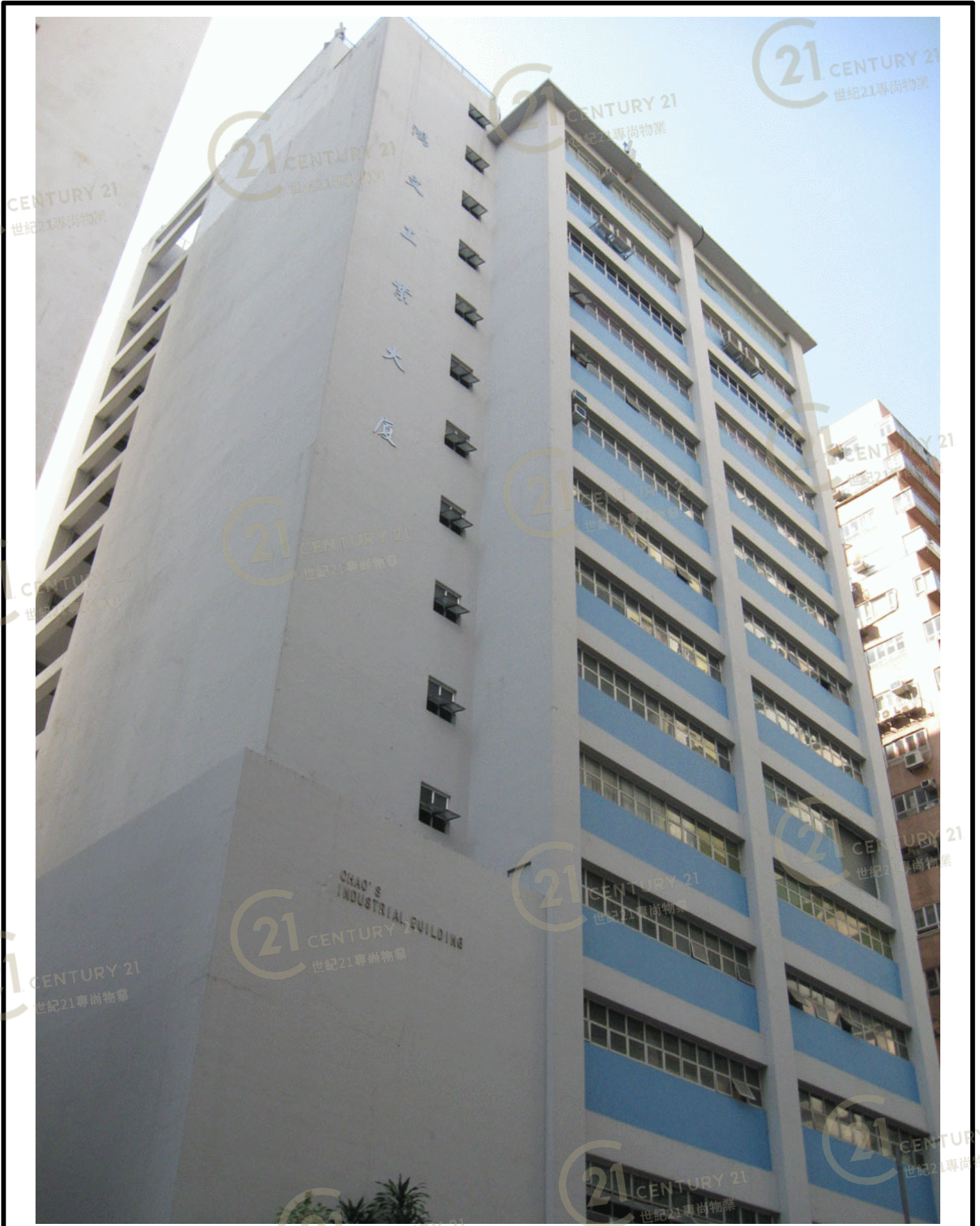
鴻文工業大廈 Chaos Industrial Building
