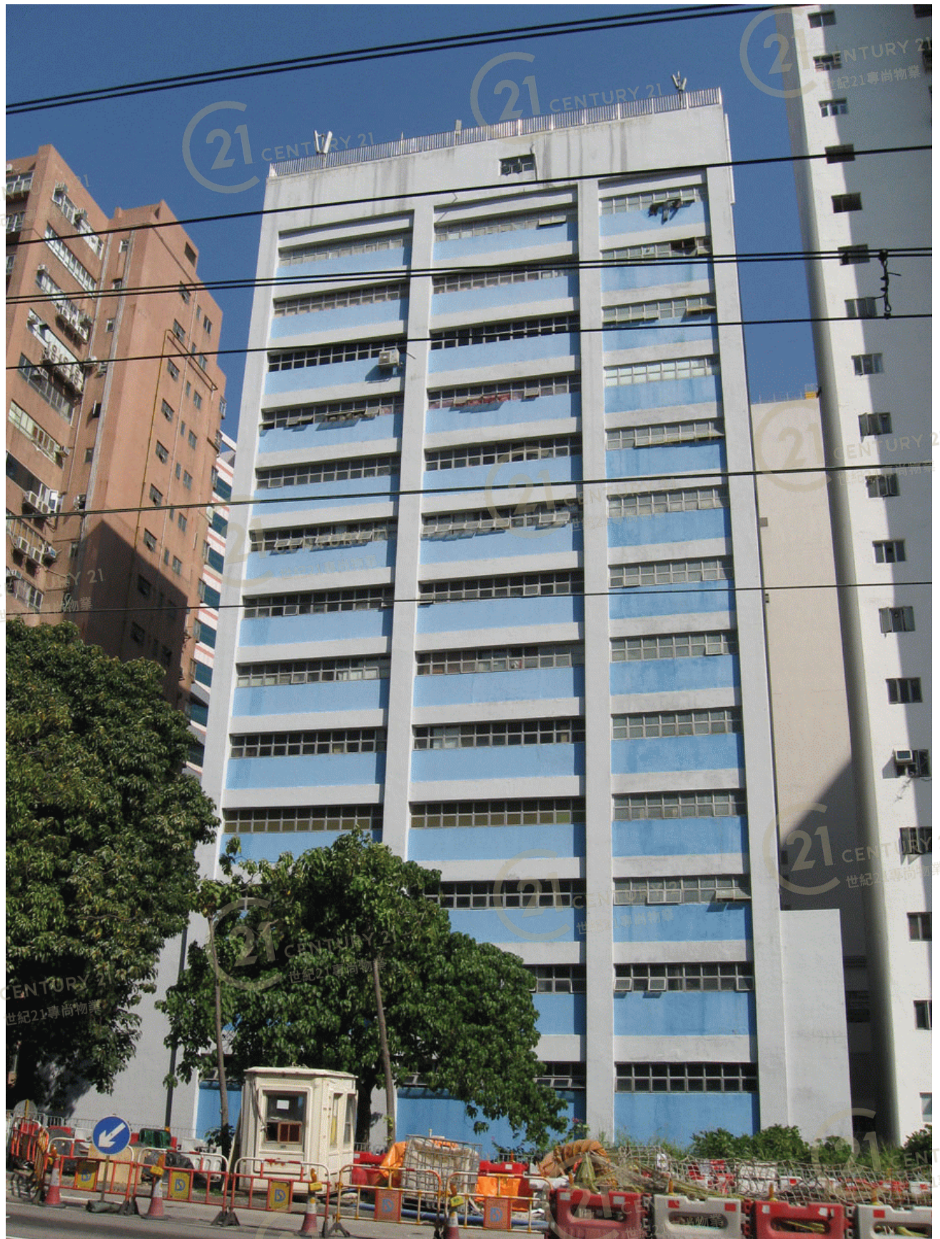
鴻文工業大廈 Chaos Industrial Building
