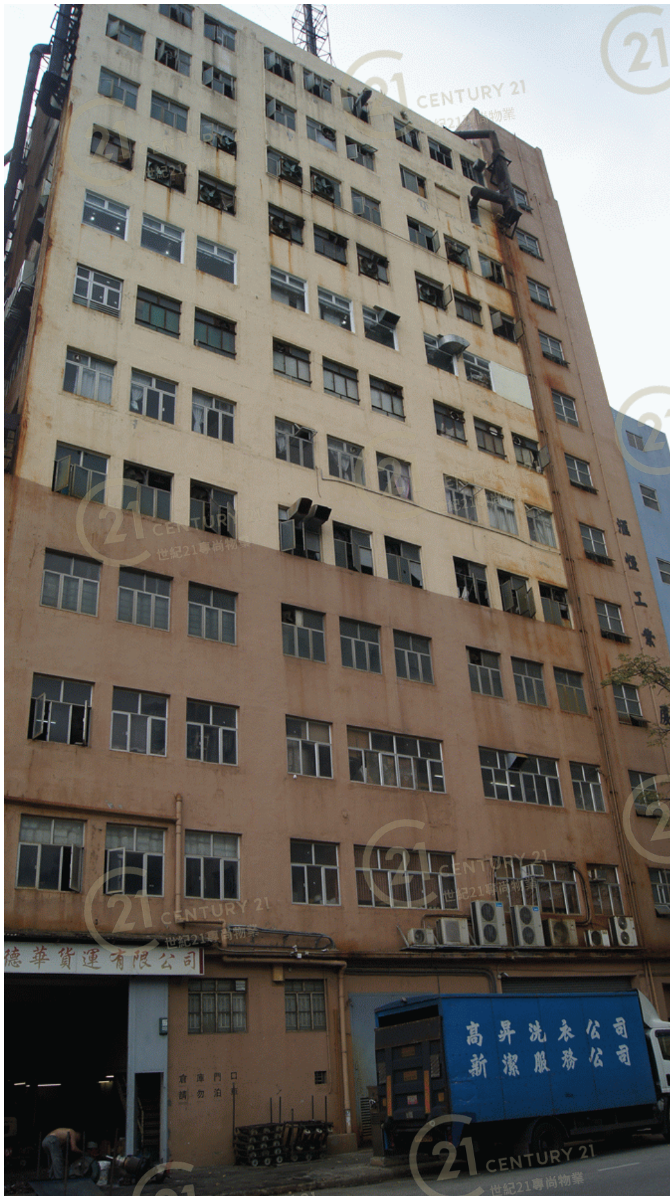
匯恒工業大廈 Hanway Industrial Building
