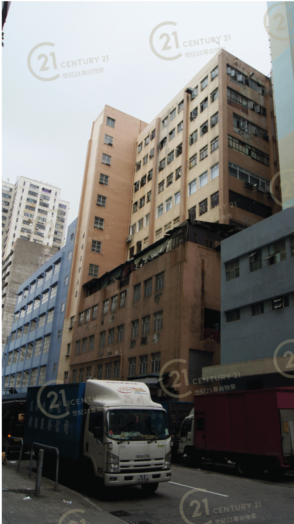
匯恒工業大廈 Hanway Industrial Building
