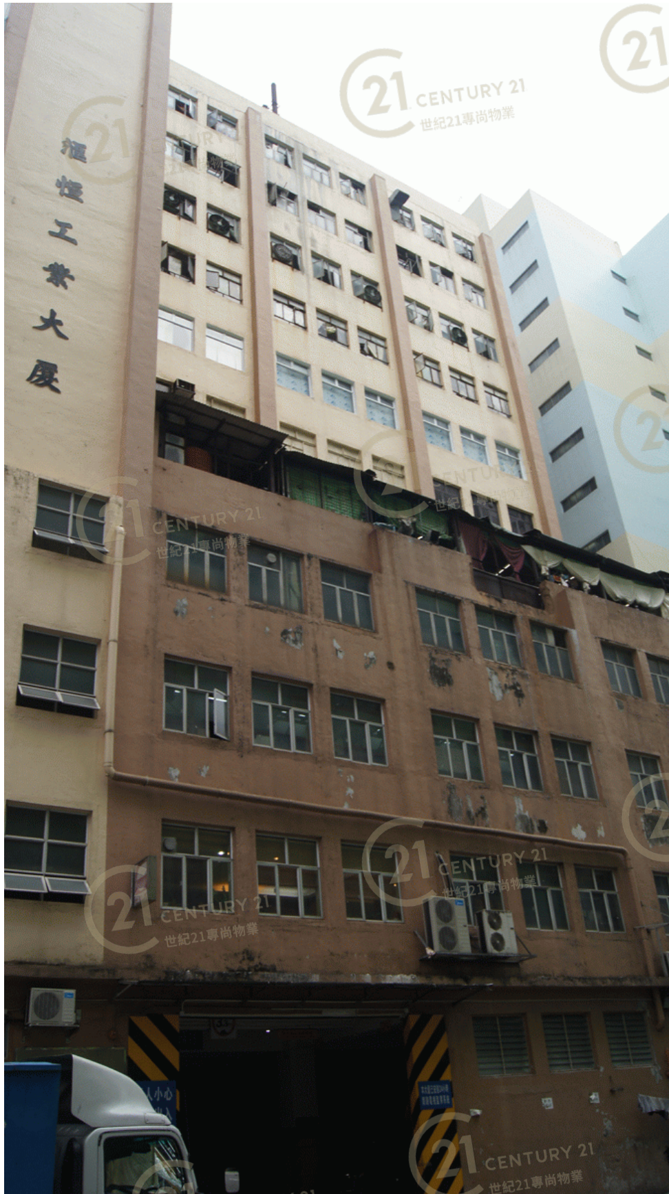
匯恒工業大廈 Hanway Industrial Building
