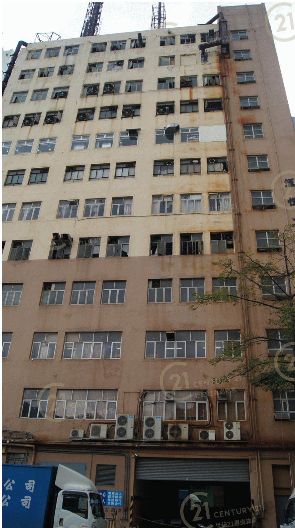
匯恒工業大廈 Hanway Industrial Building
