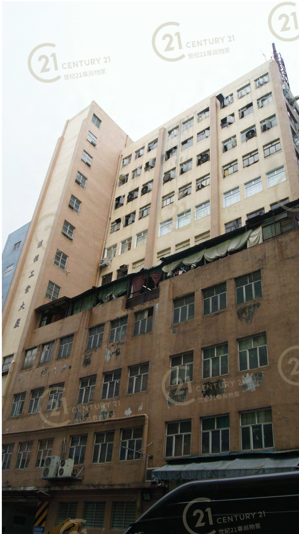
匯恒工業大廈 Hanway Industrial Building
