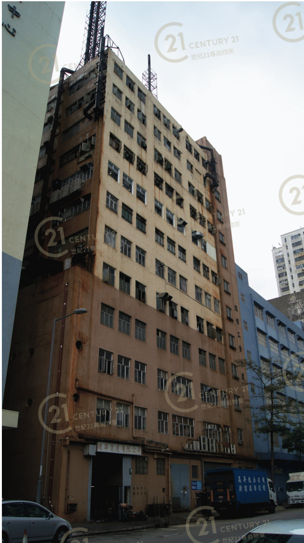
匯恒工業大廈 Hanway Industrial Building
