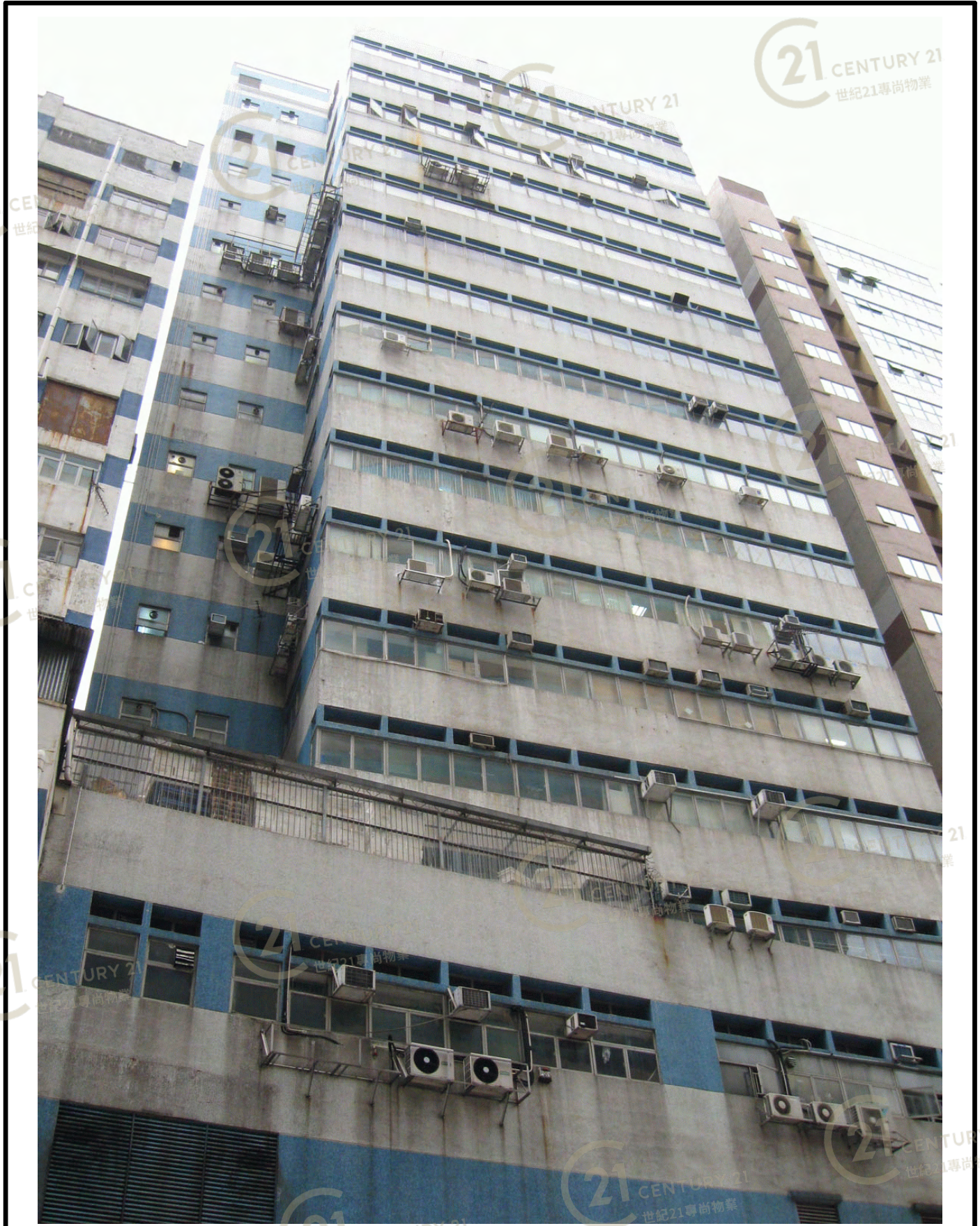
葵匯工業大廈 Kwai Wu Industrial Building
