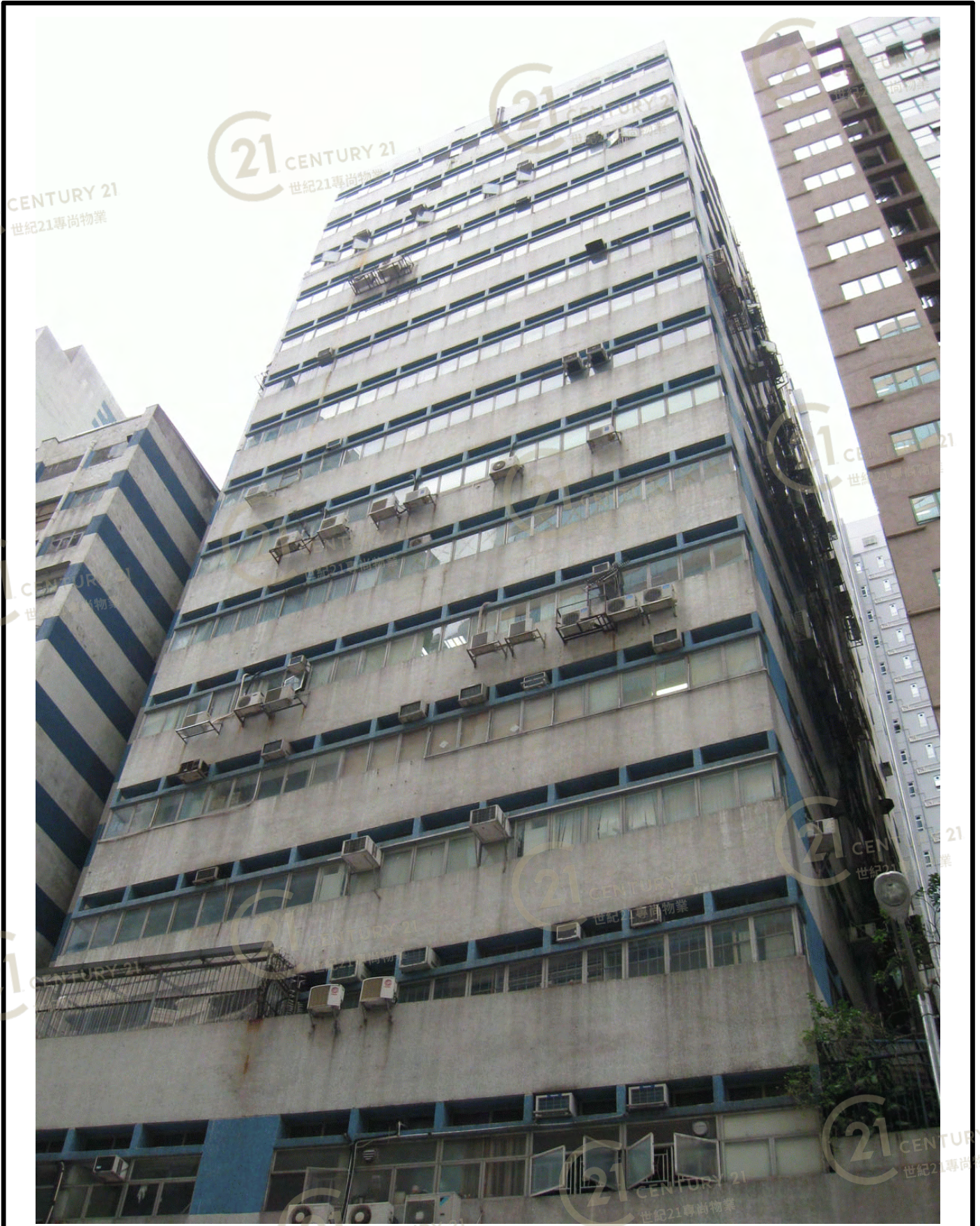
葵匯工業大廈 Kwai Wu Industrial Building
