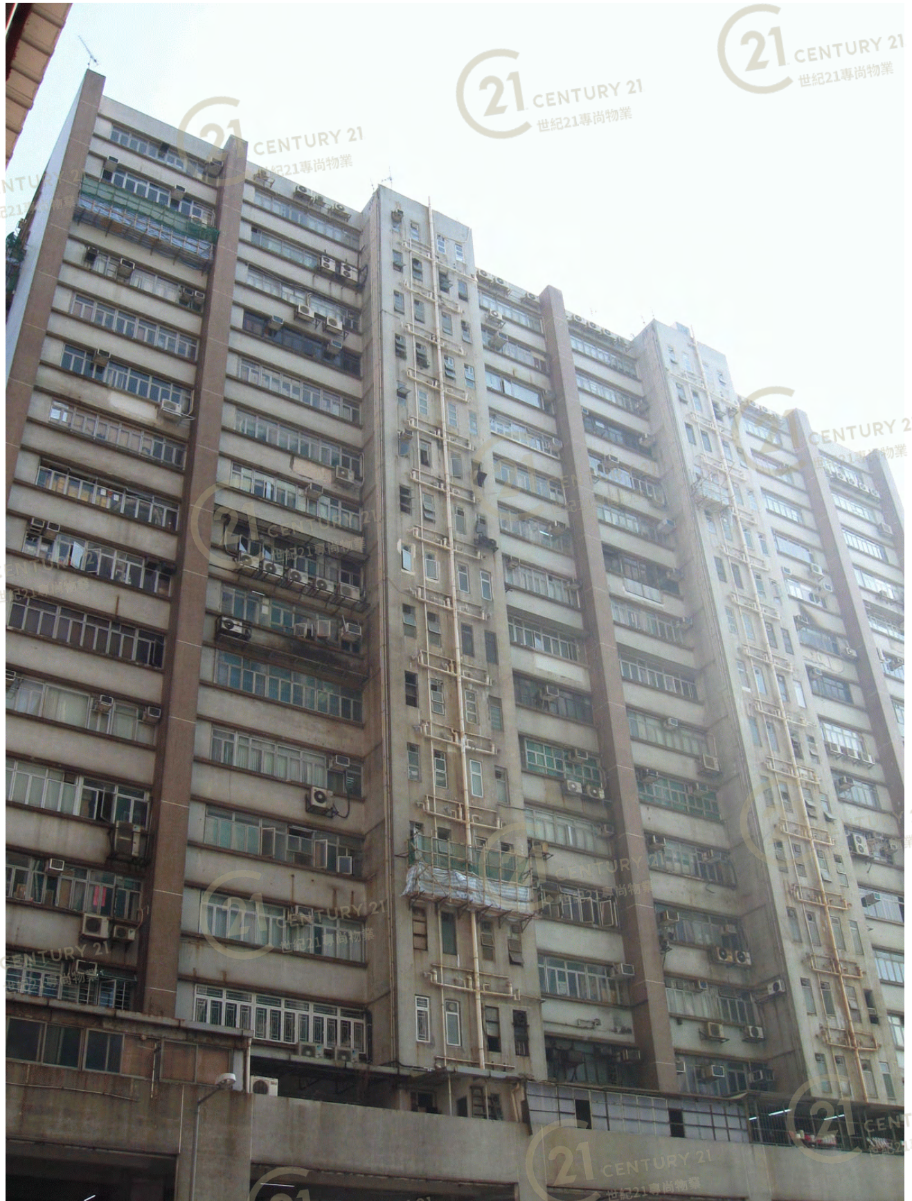
永恒工業大廈 Wing Hang Industrial Building
