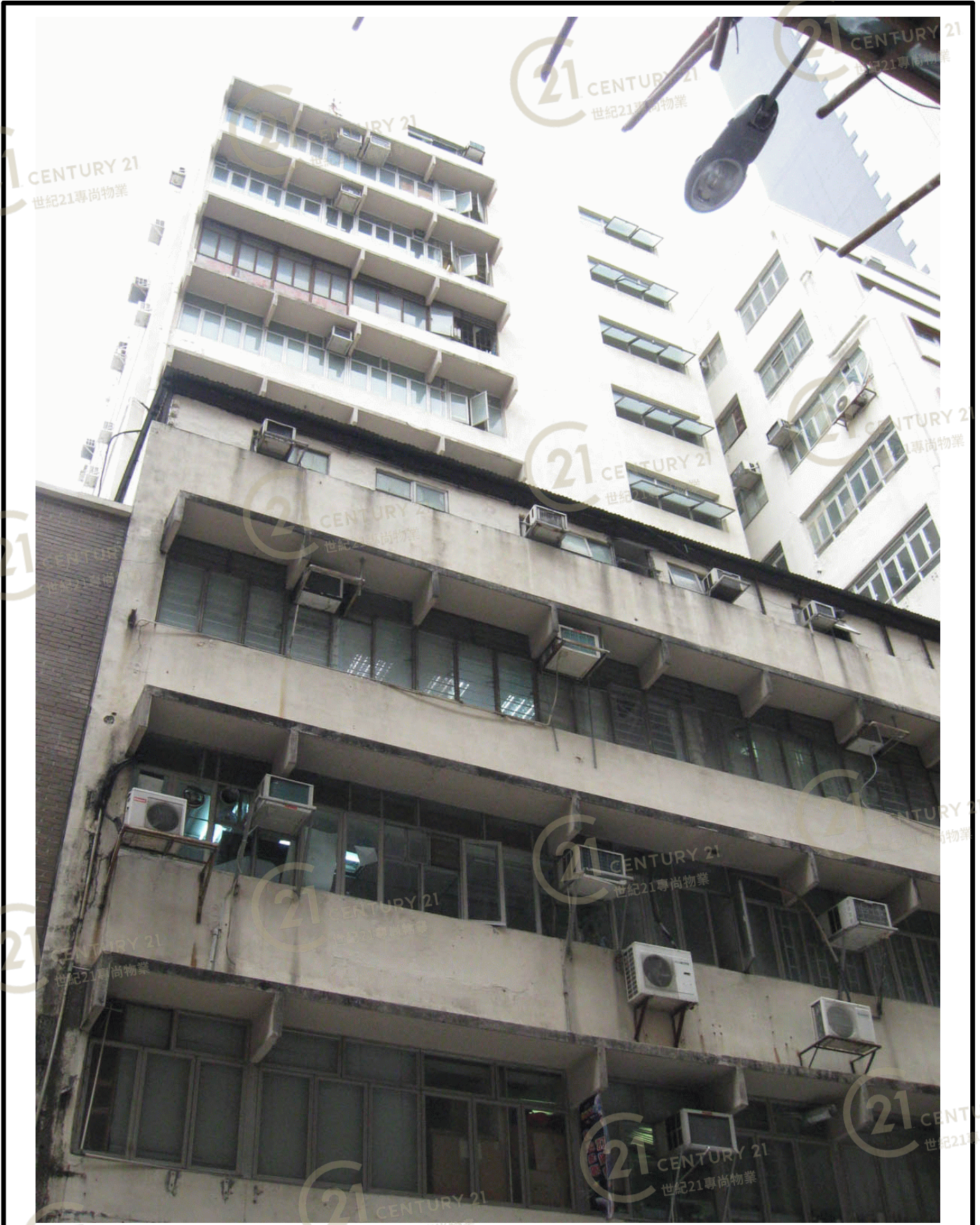
中溪工業大廈 Chung Kai Factory Building
