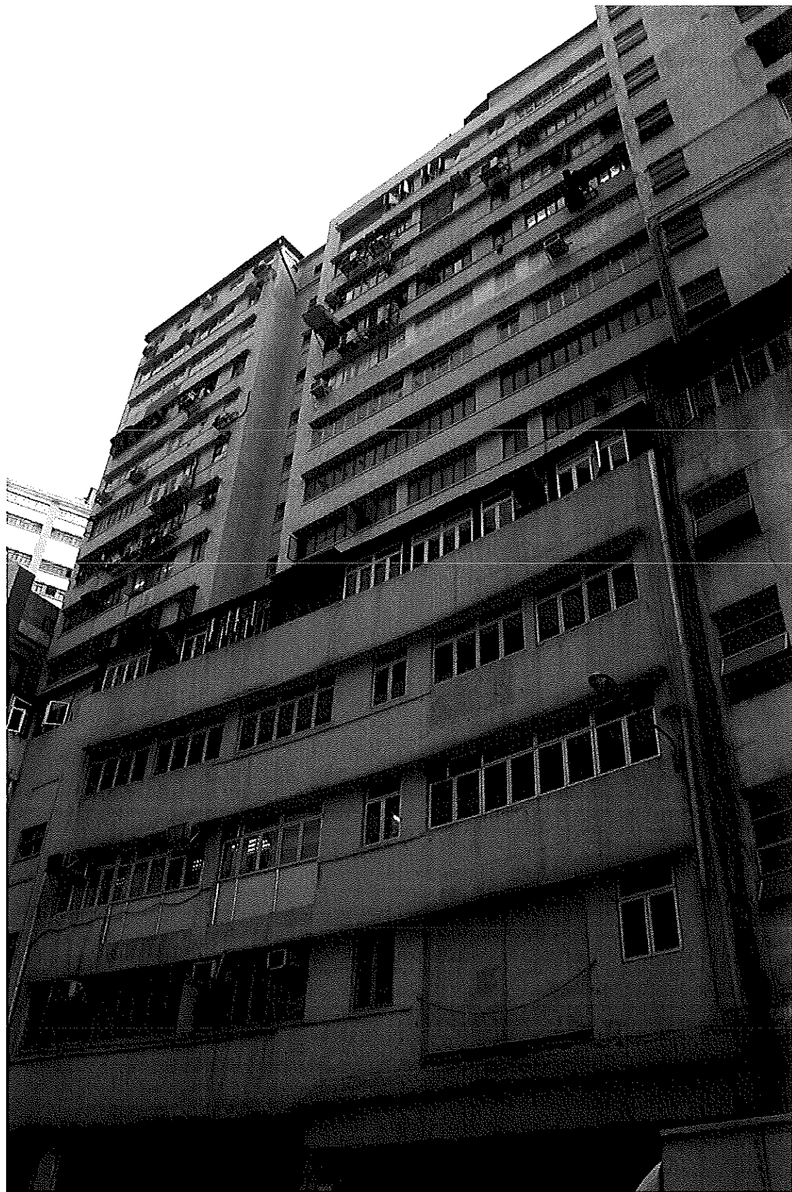
華興工業大廈 (荃灣) Wah Hing Industrial Building (TW)
