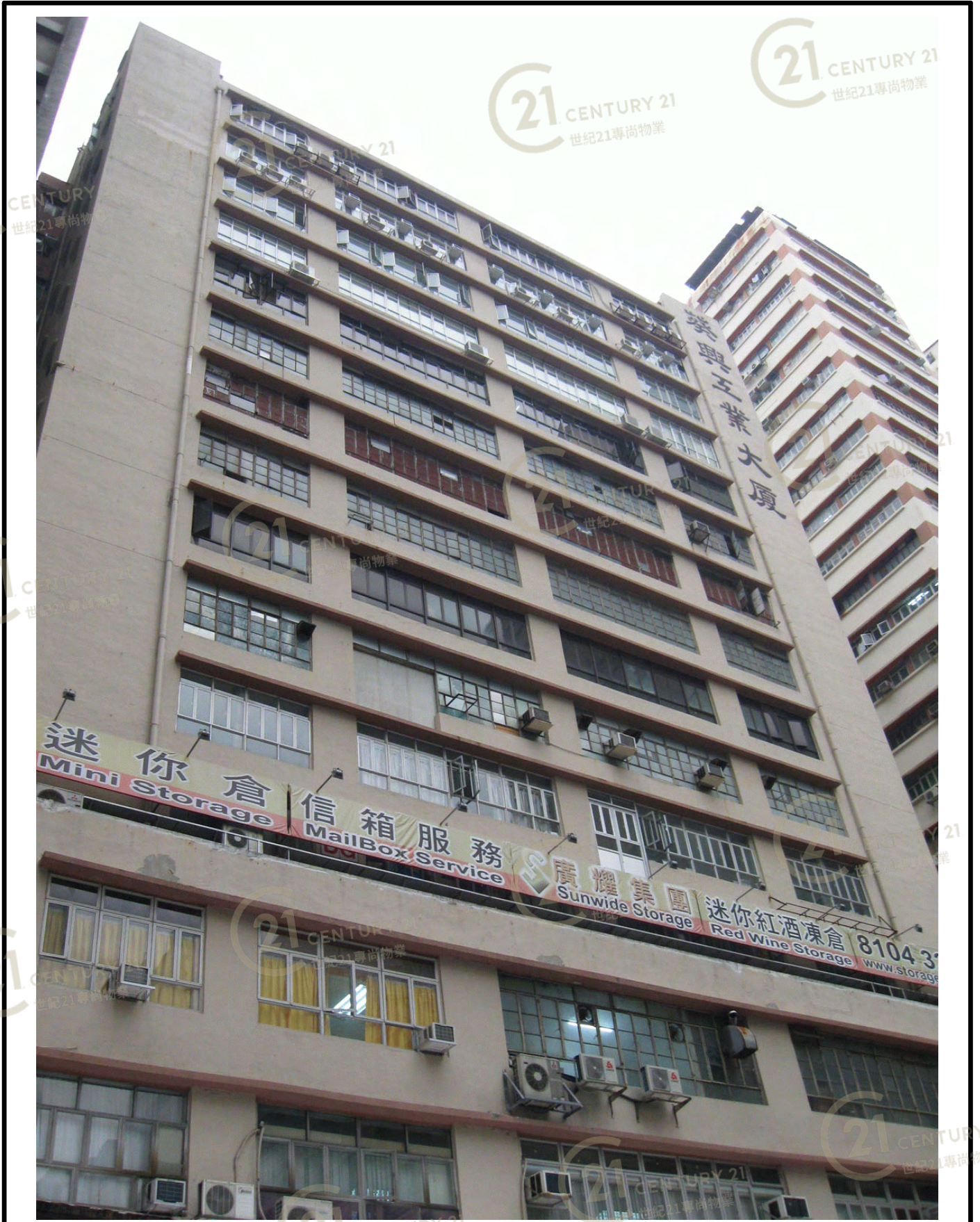
葵興工業大廈 Kwai Hing Industrial Building
