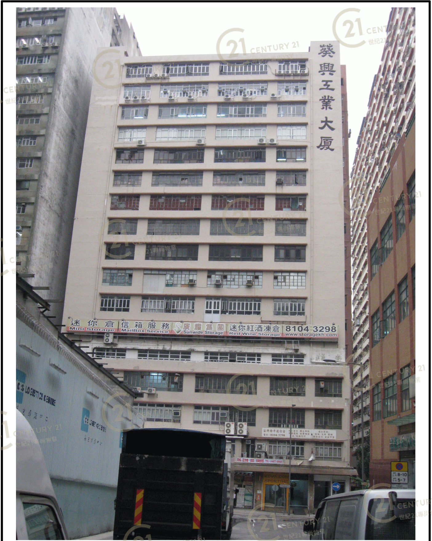
葵興工業大廈 Kwai Hing Industrial Building
