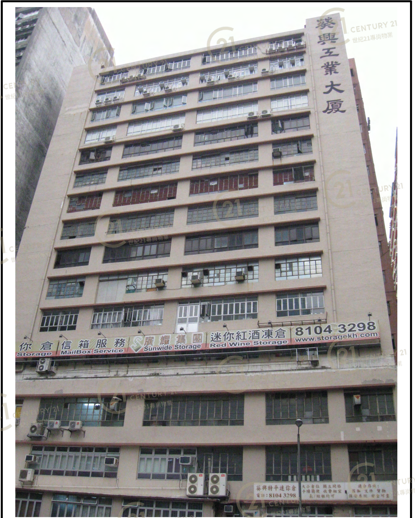
葵興工業大廈 Kwai Hing Industrial Building
