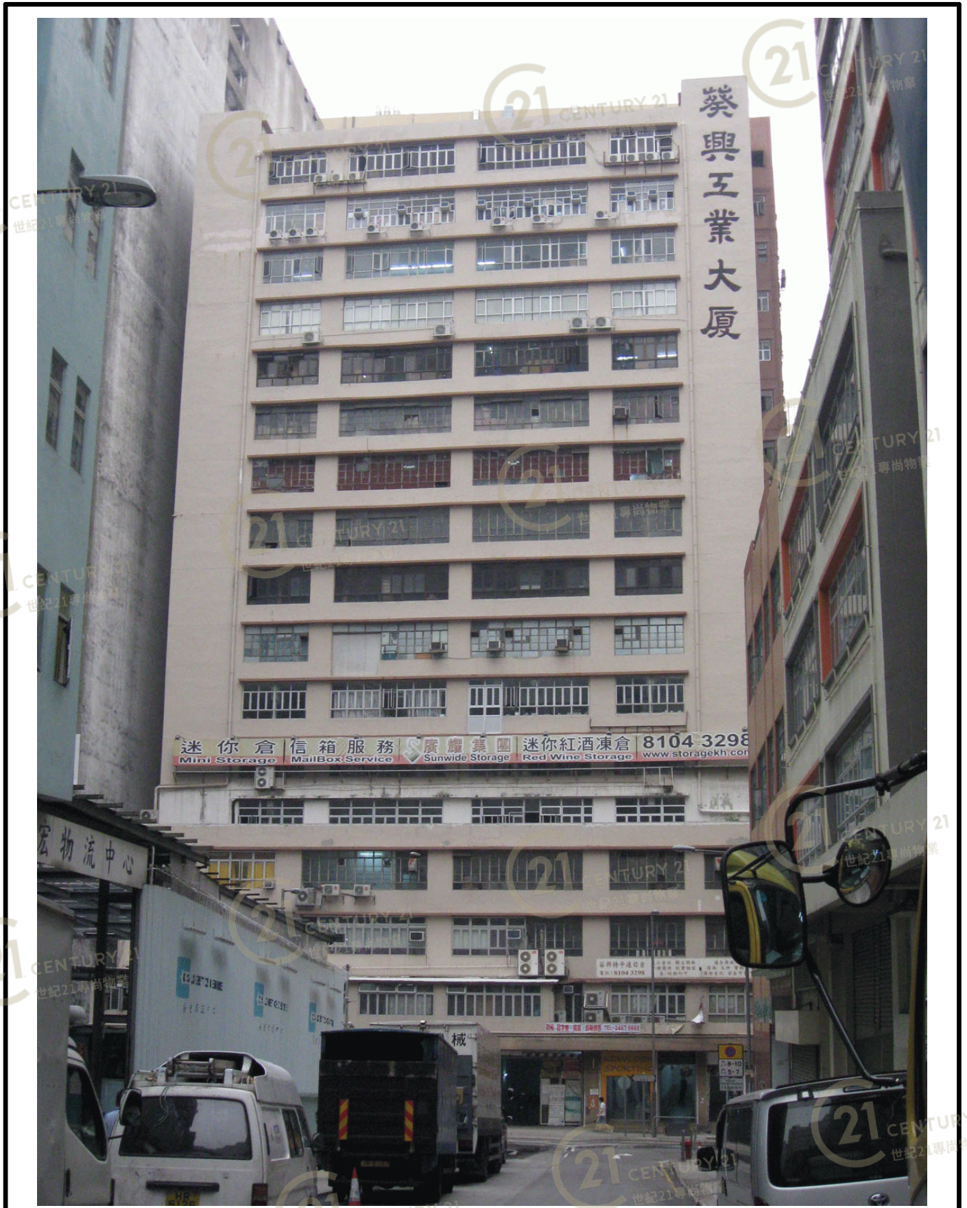
葵興工業大廈 Kwai Hing Industrial Building
