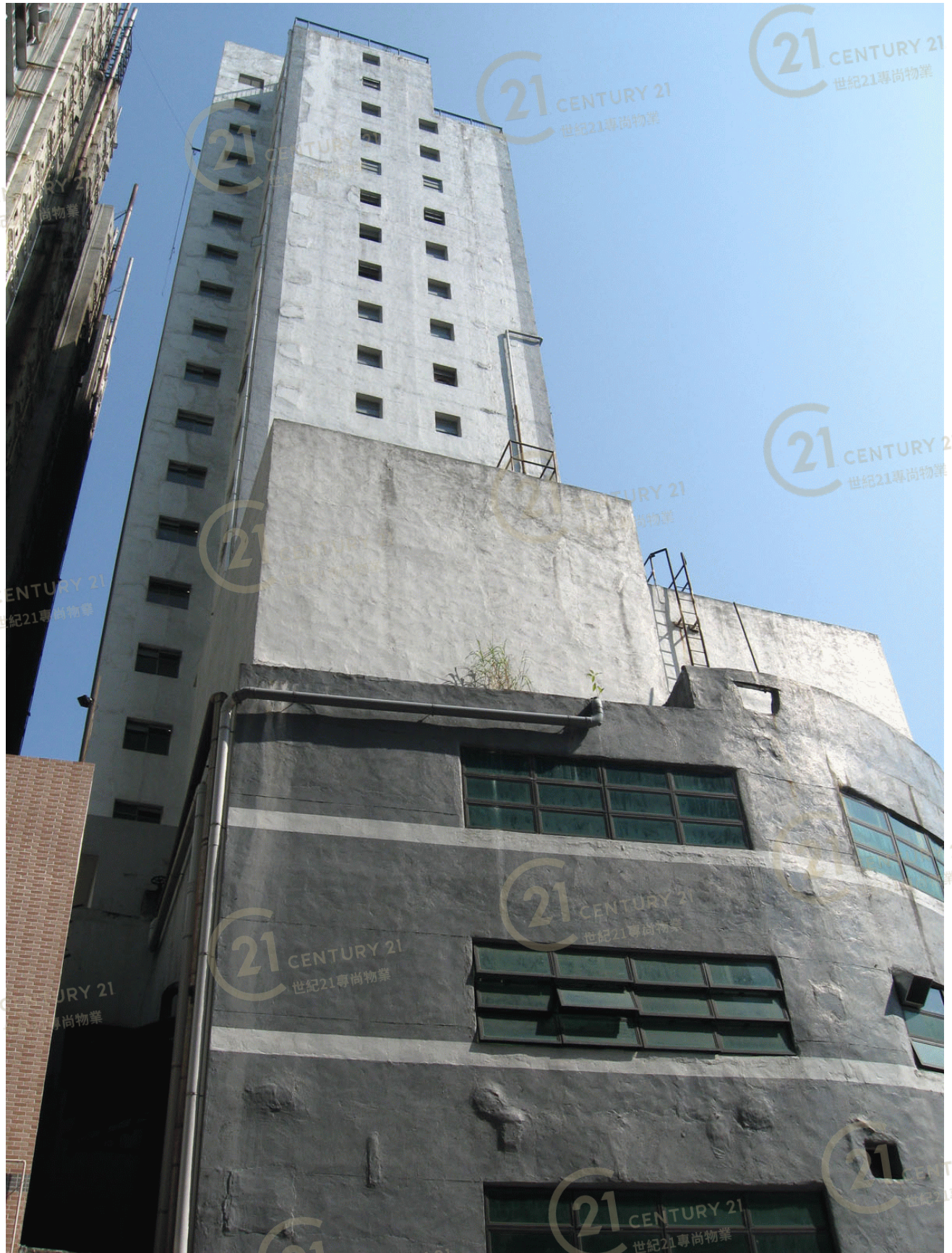
葵灣工業大廈 Kwai Wan Industrial Building
