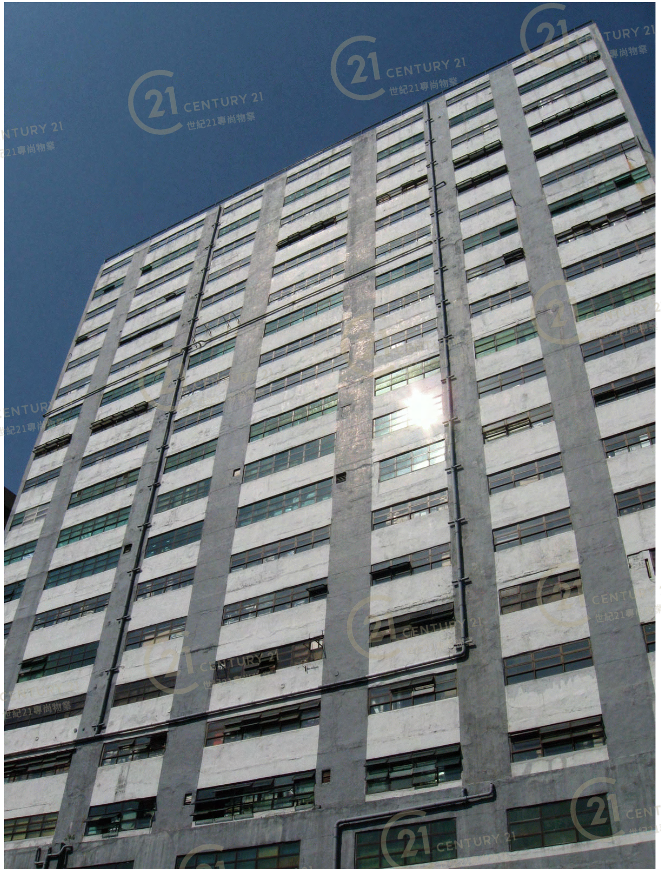
葵灣工業大廈 Kwai Wan Industrial Building
