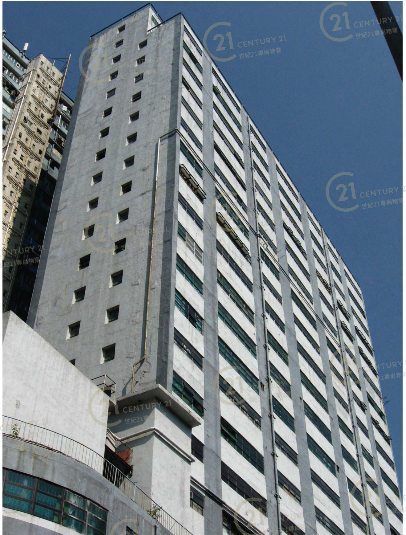
葵灣工業大廈 Kwai Wan Industrial Building
