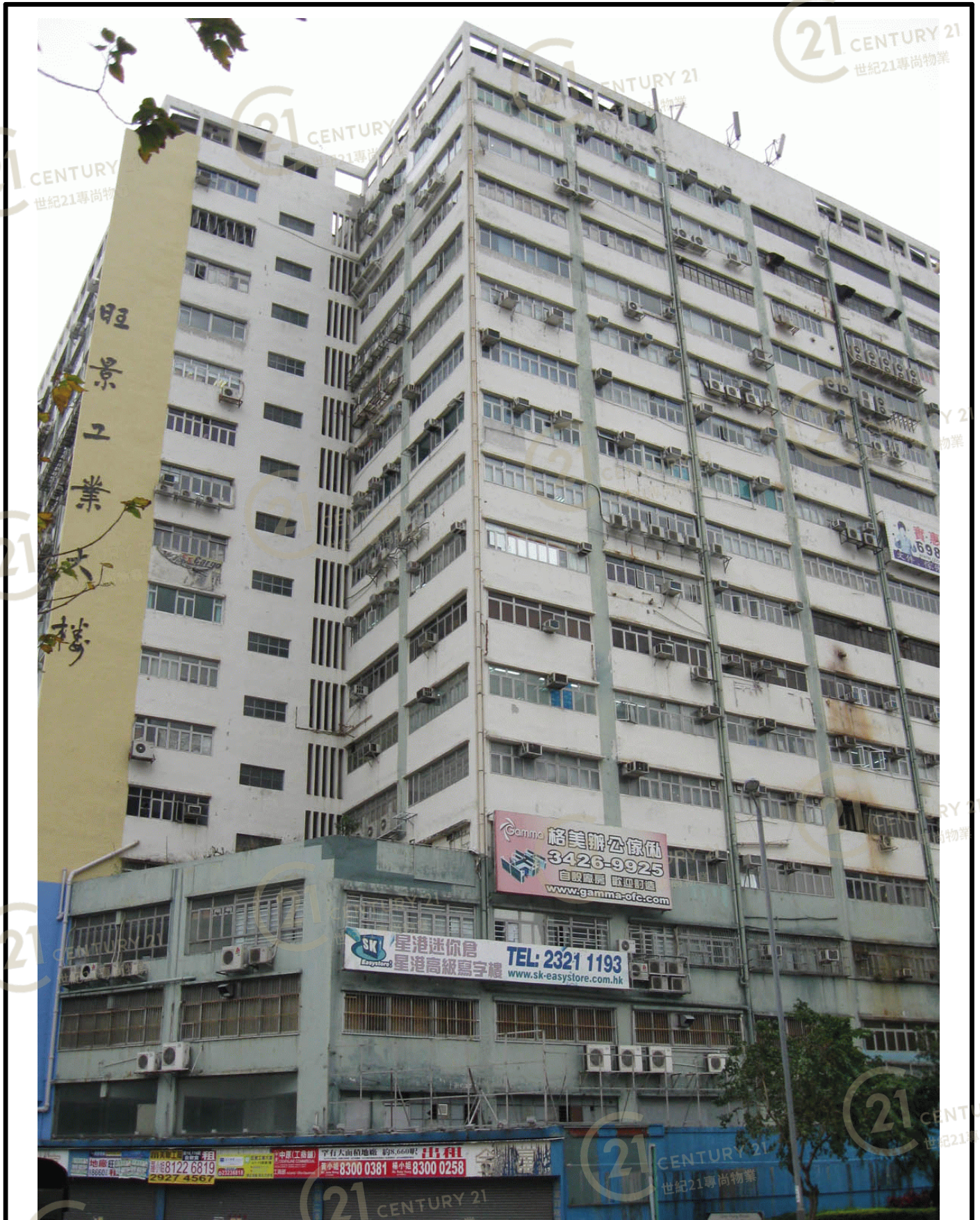
旺景工業大廈 Wong King Industrial Building
