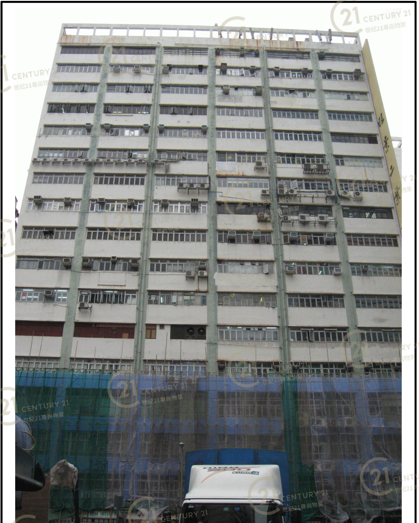
旺景工業大廈 Wong King Industrial Building
