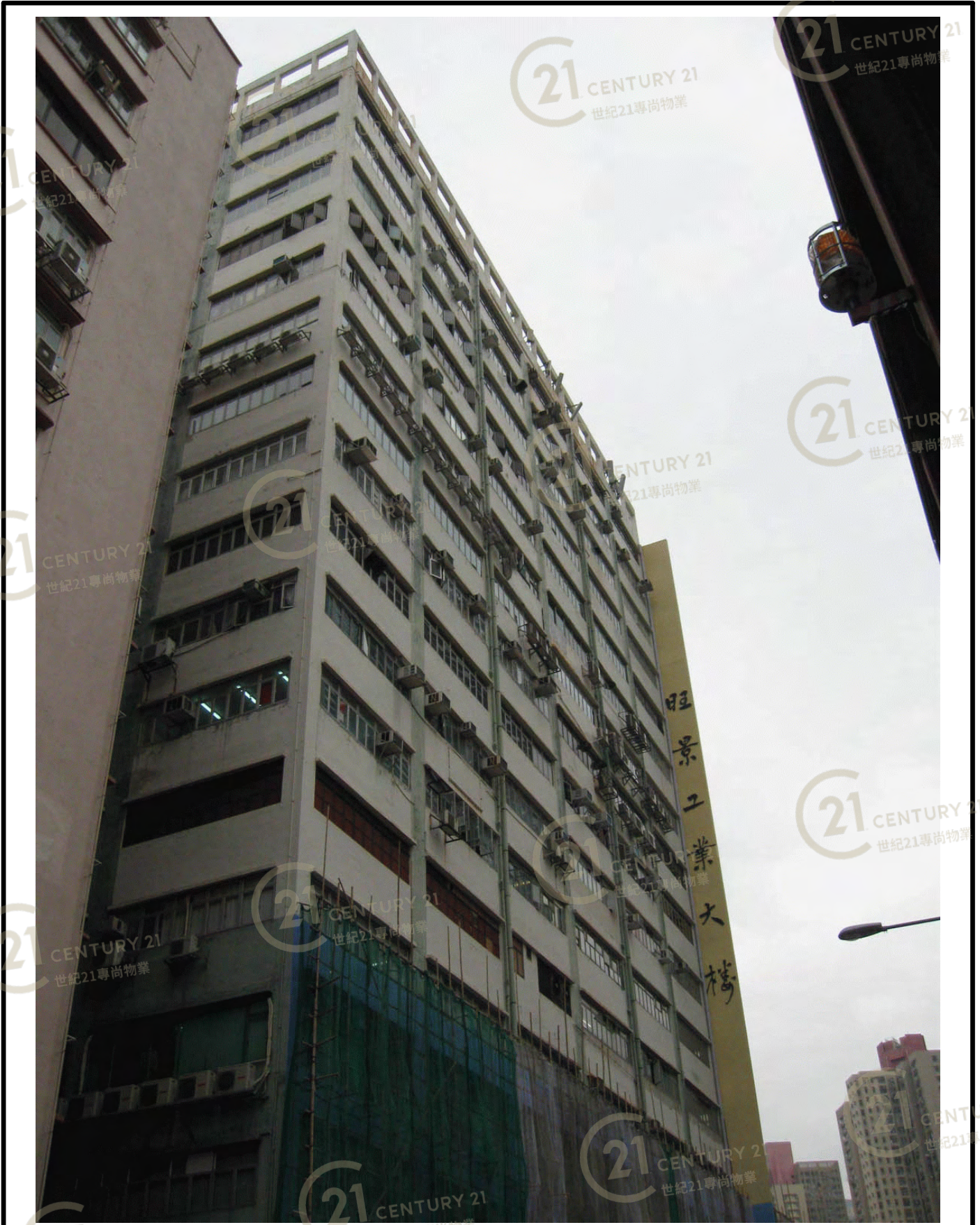
旺景工業大廈 Wong King Industrial Building
