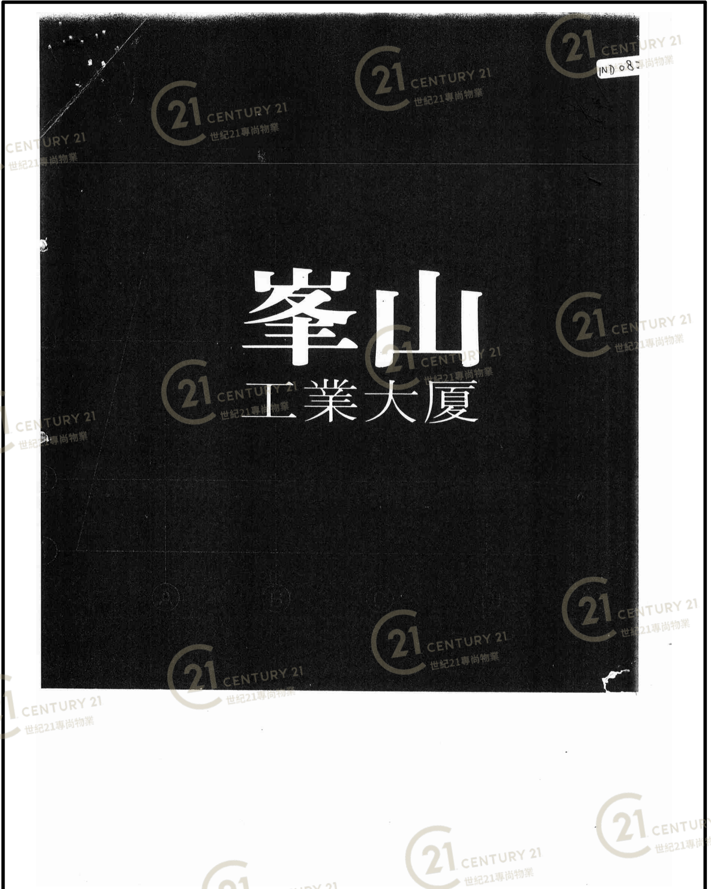
峰山工業大廈 Supreme Industrial Building
