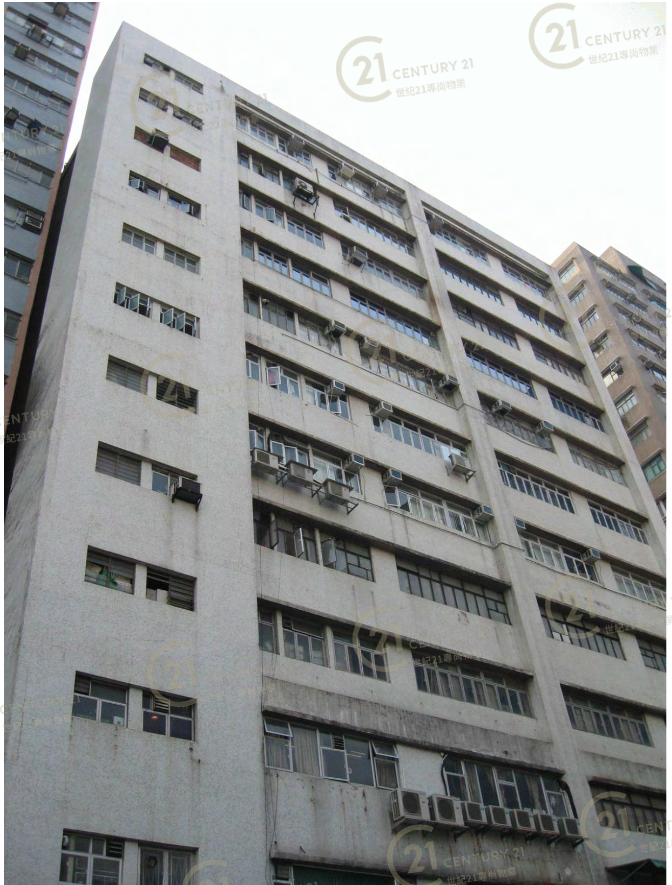
峰山工業大廈 Supreme Industrial Building
