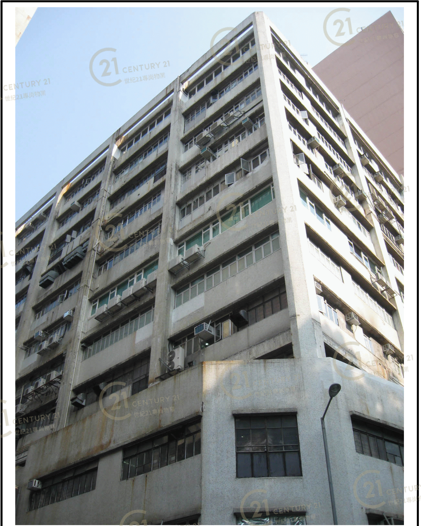
峰山工業大廈 Supreme Industrial Building
