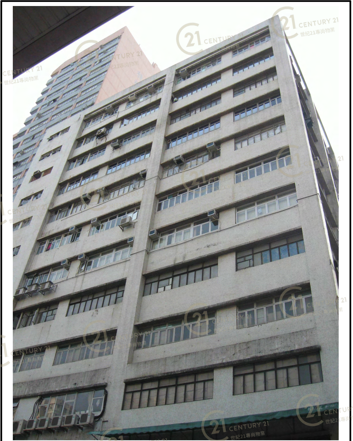
峰山工業大廈 Supreme Industrial Building
