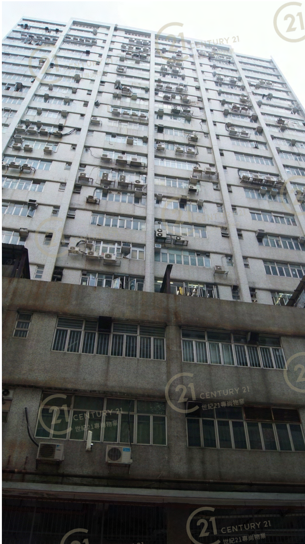
建榮工業大廈 Kin Wing Industrial Building
