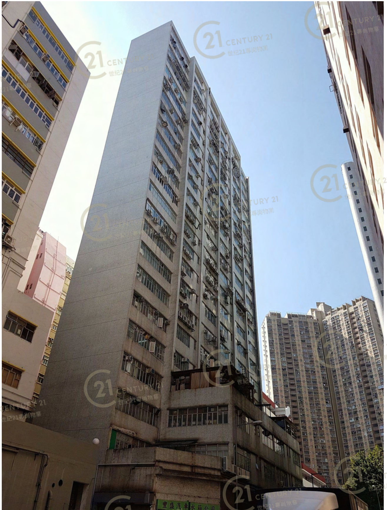
建榮工業大廈 Kin Wing Industrial Building
