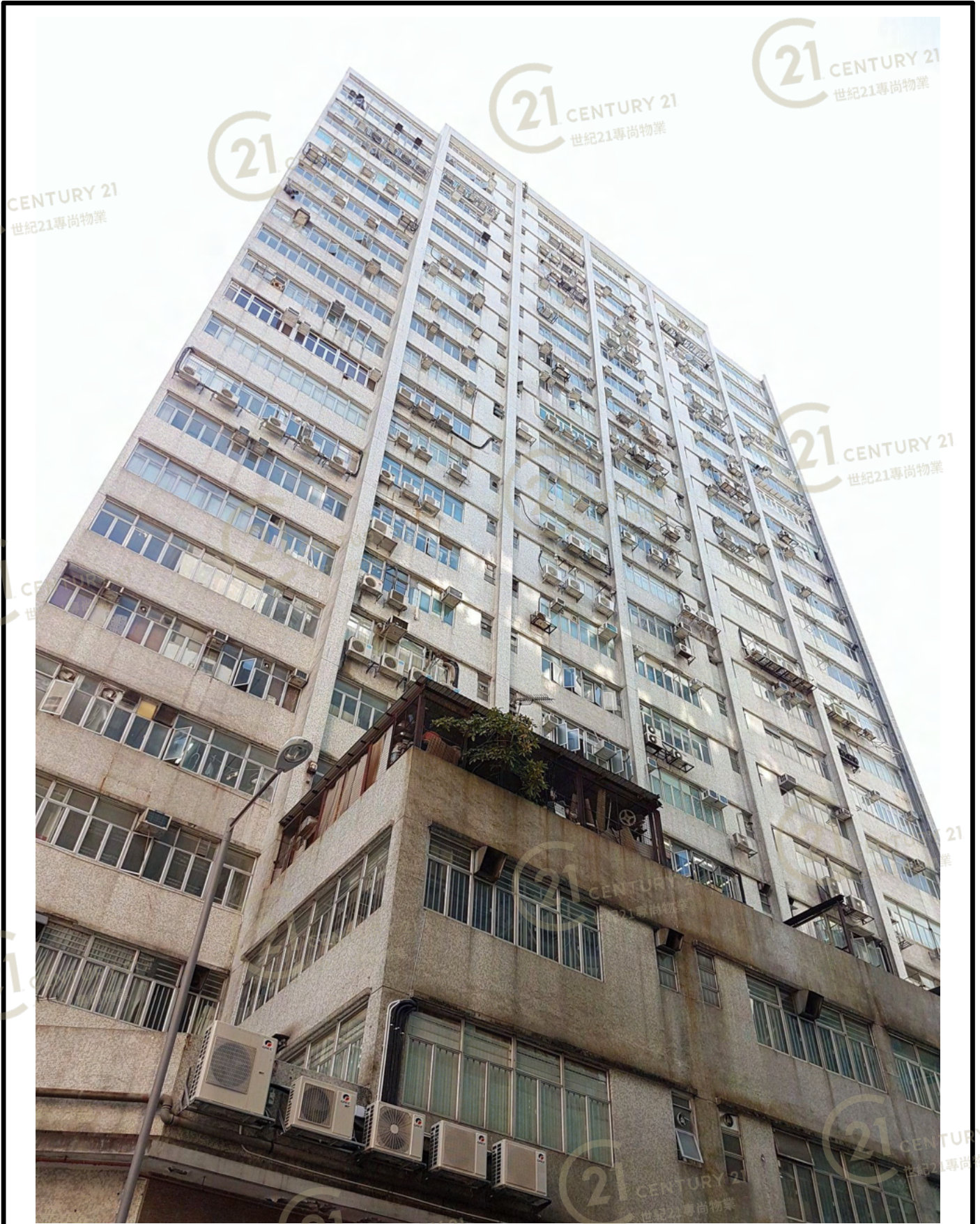
建榮工業大廈 Kin Wing Industrial Building
