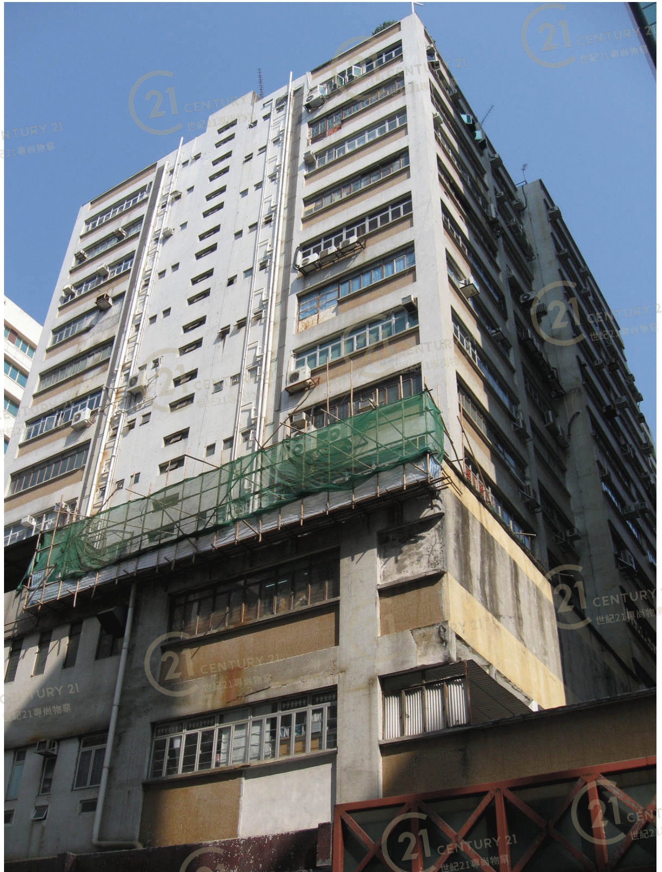
聯邦工業大廈 Leapont Industrial Building
