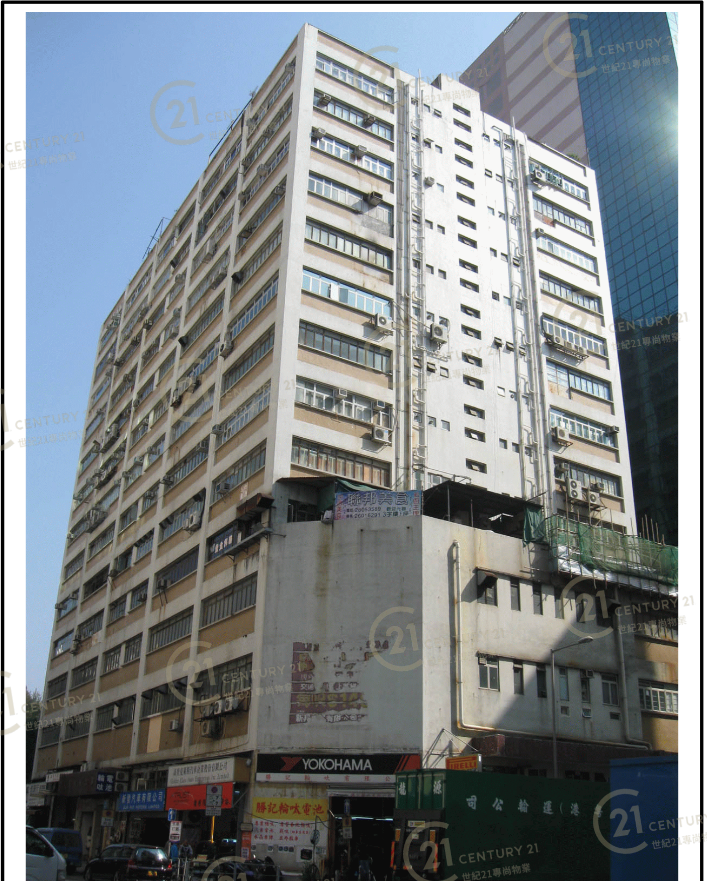
聯邦工業大廈 Leapont Industrial Building
