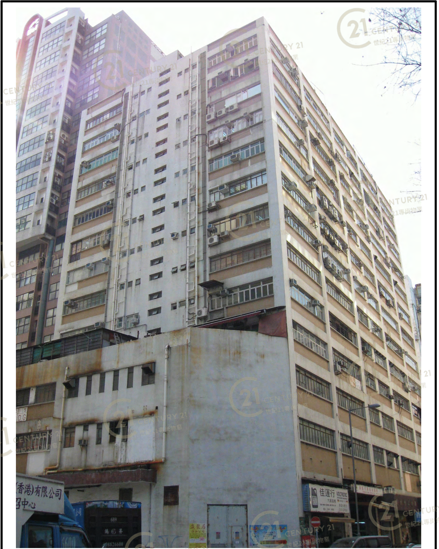
聯邦工業大廈 Leapont Industrial Building
