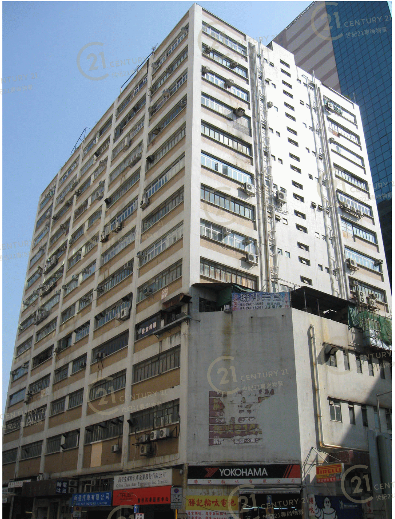
聯邦工業大廈 Leapont Industrial Building
