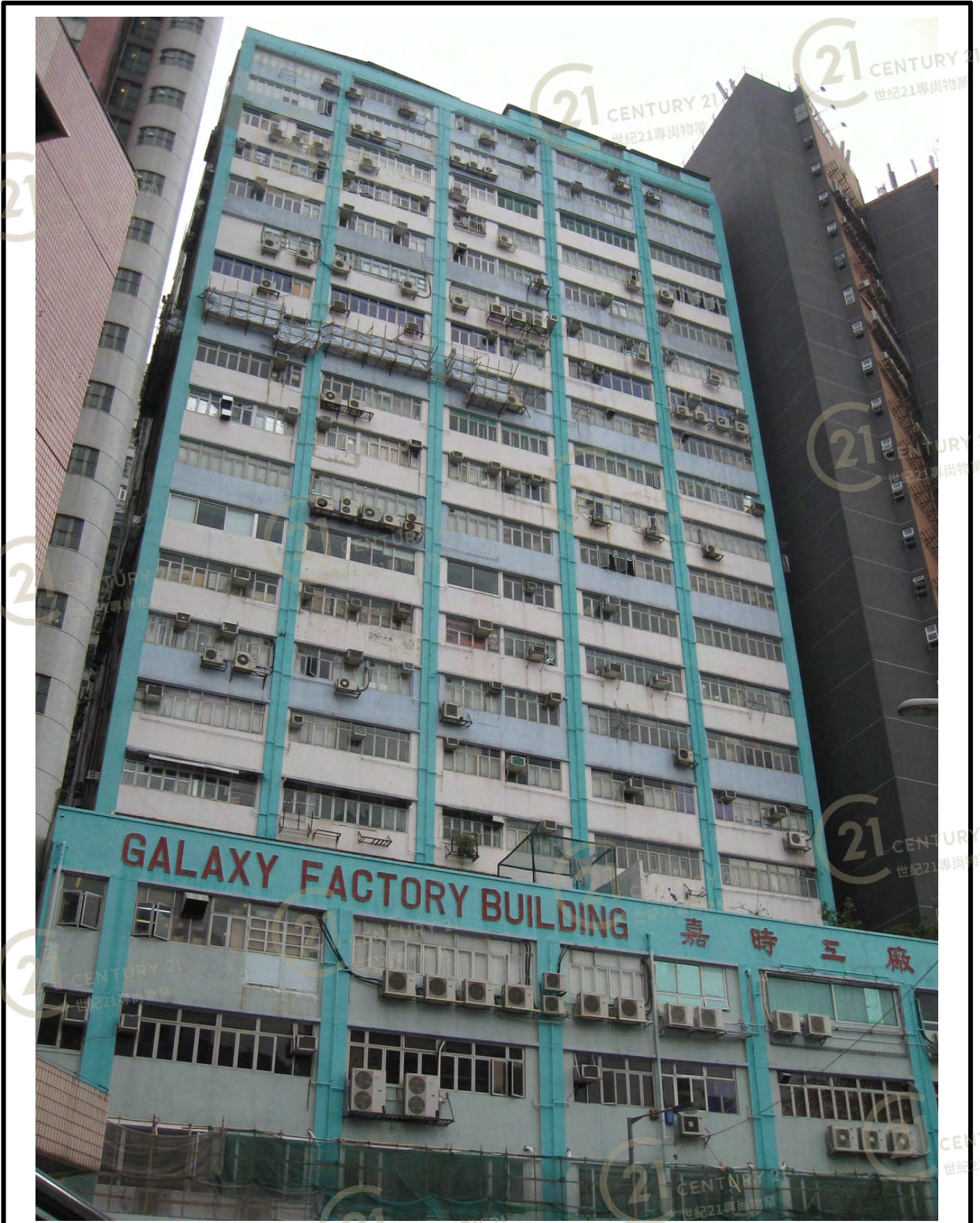
嘉時工廠大廈 Galaxy Factory Building
