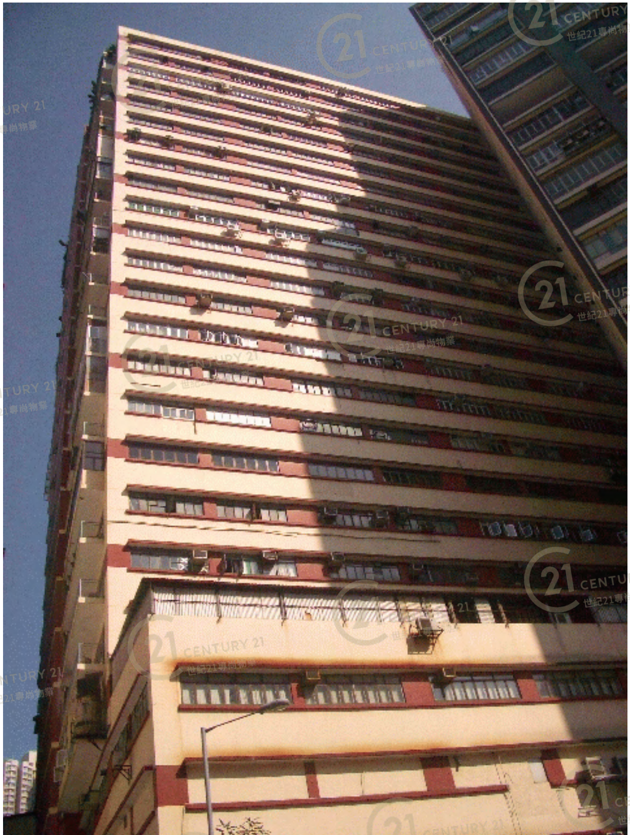
保盈工業大廈 Bold Win Industrial Building
