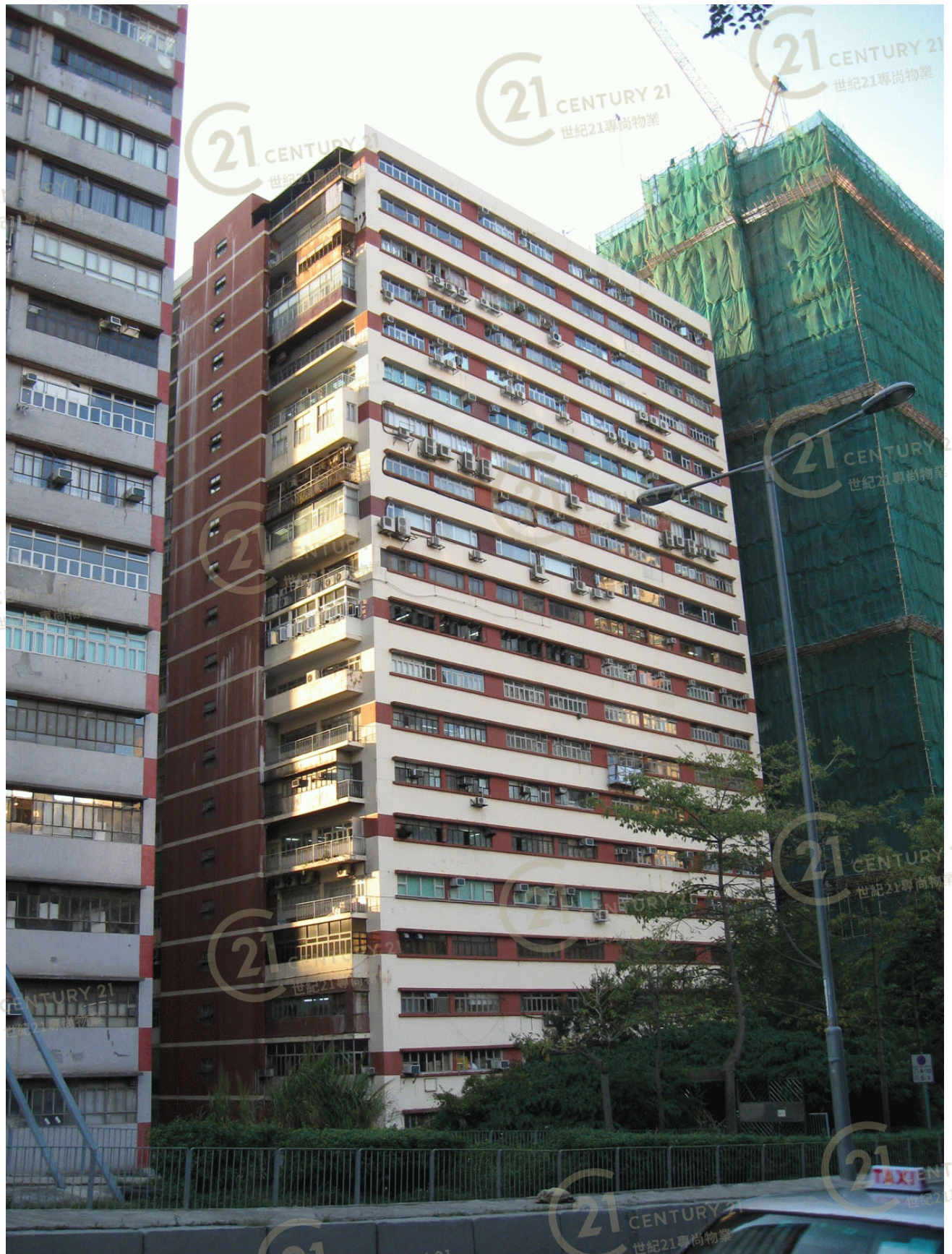
保盈工業大廈 Bold Win Industrial Building
