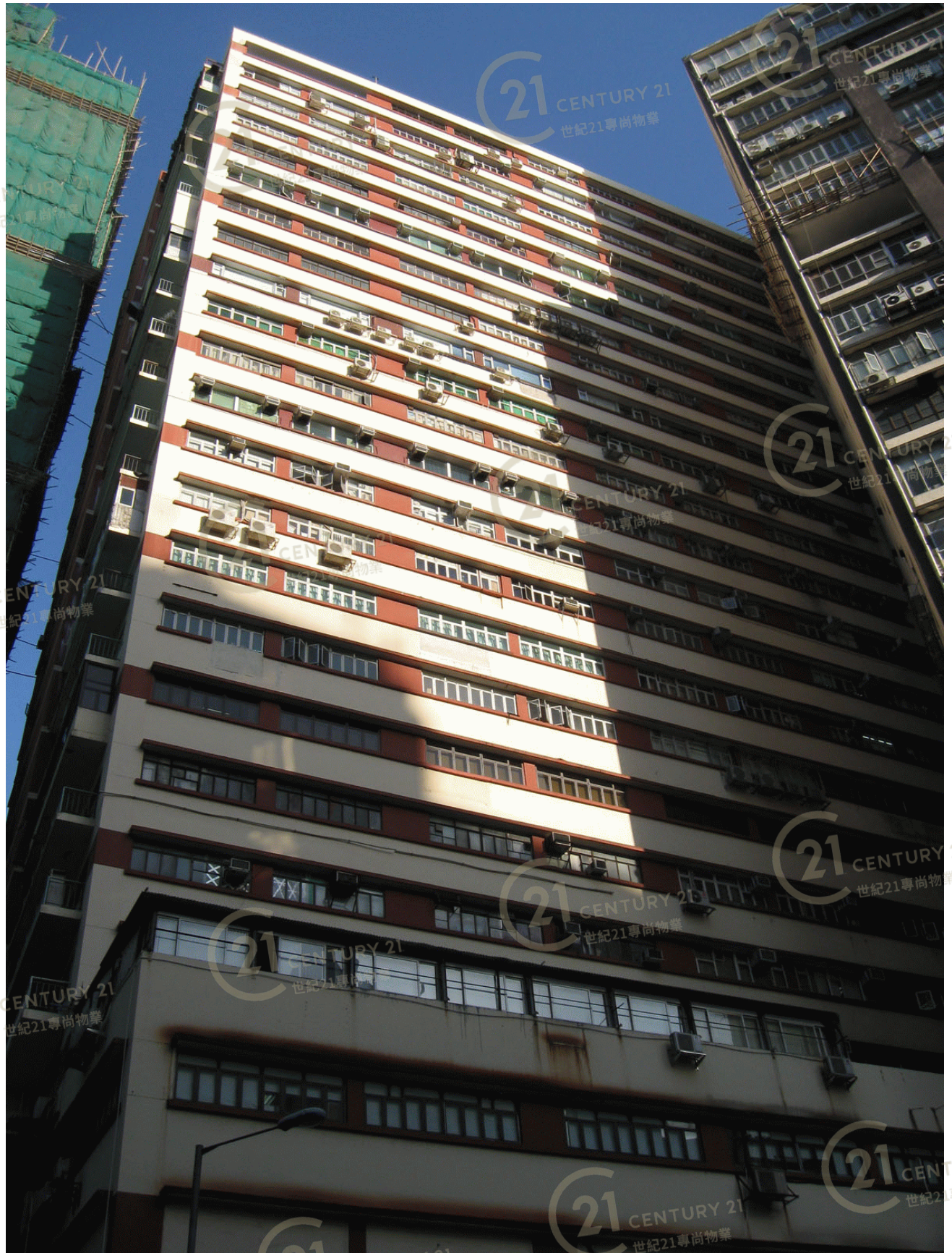
保盈工業大廈 Bold Win Industrial Building
