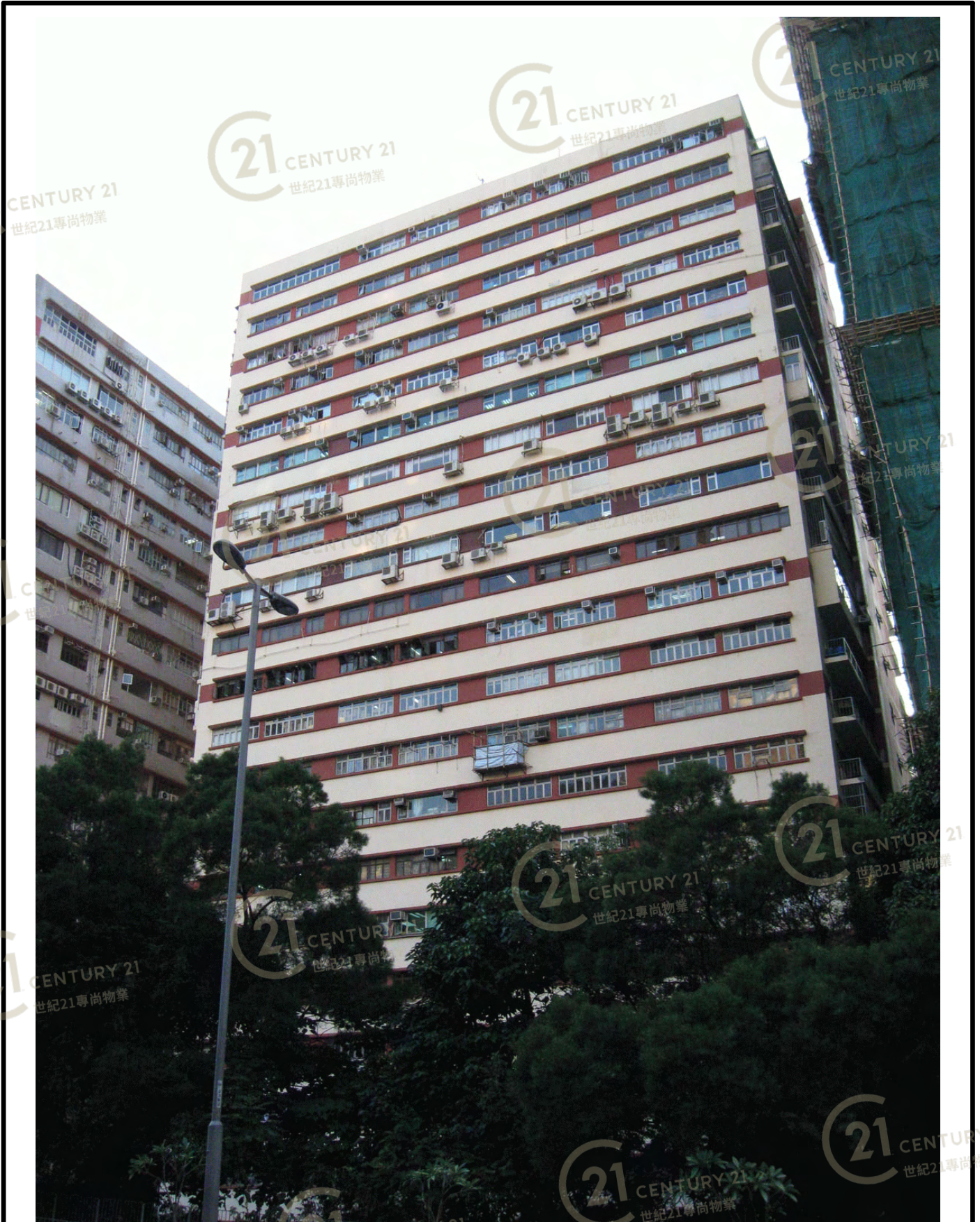
保盈工業大廈 Bold Win Industrial Building
