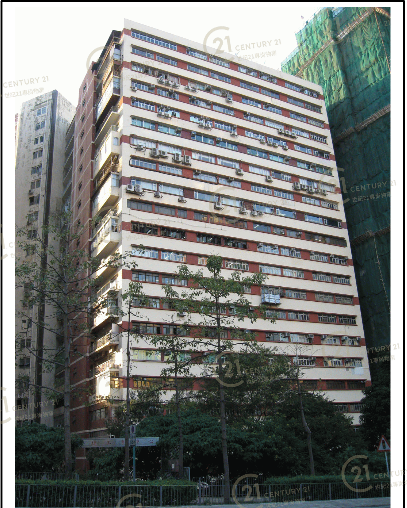
保盈工業大廈 Bold Win Industrial Building
