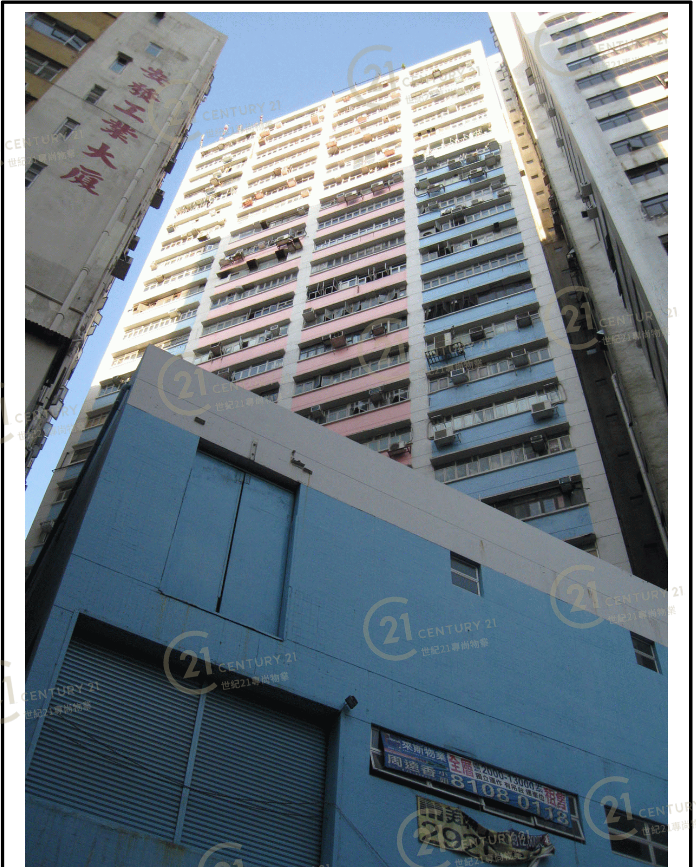
瑞森工業大廈 Shui Sum Industrial Building
