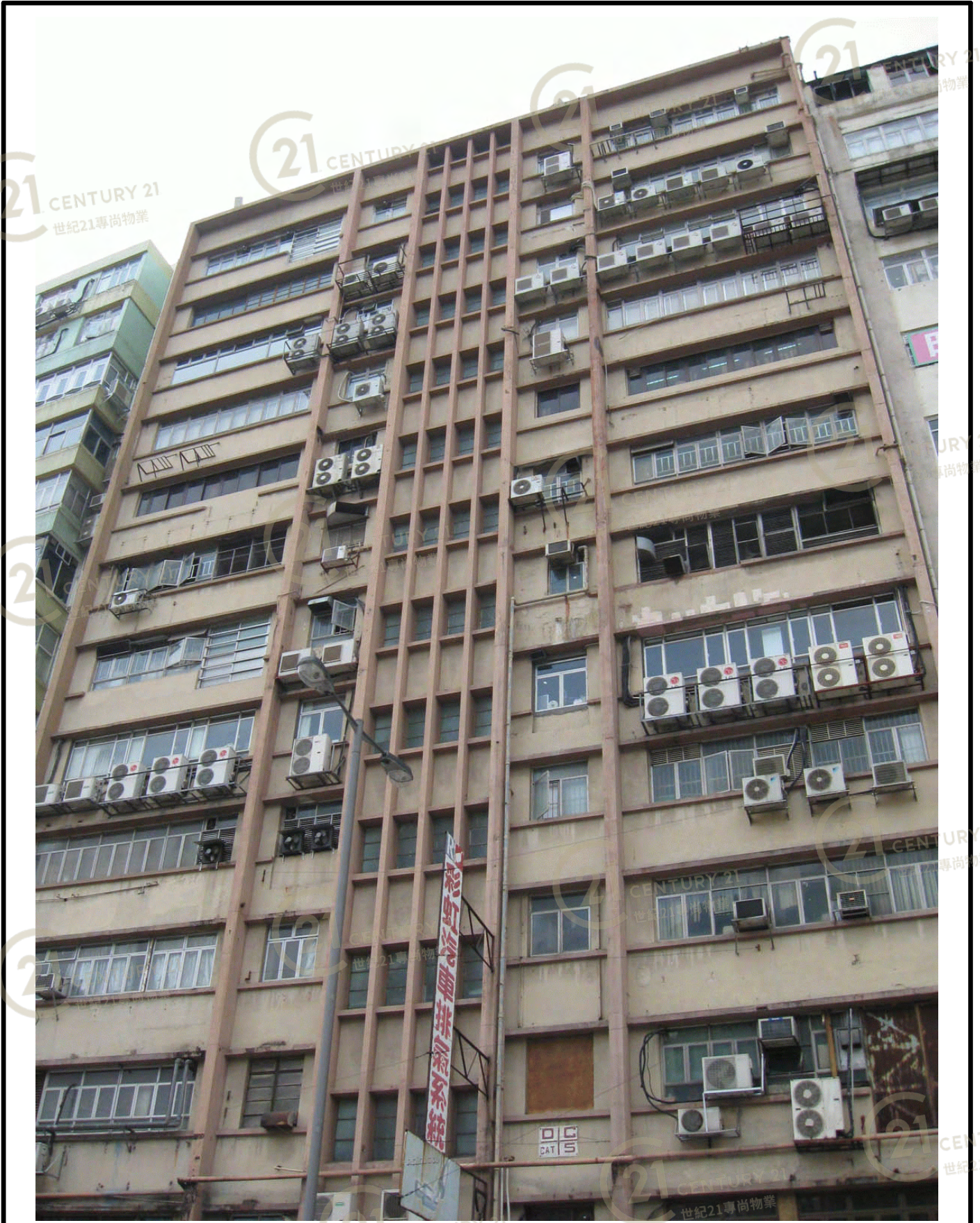
緯綸工業大廈 William Enterprises Industrial Building
