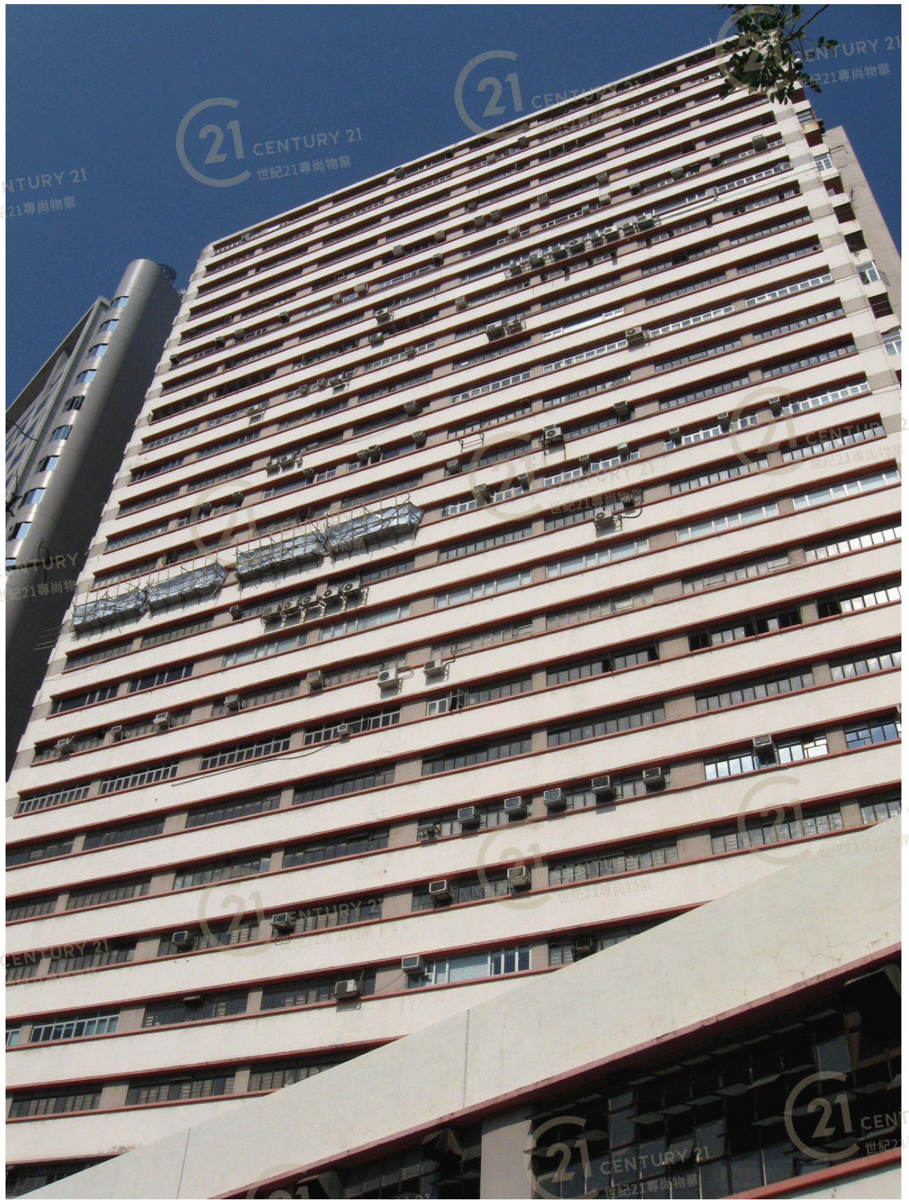
金發工業大廈1期 Kingsford Industrial Building Phase 1
