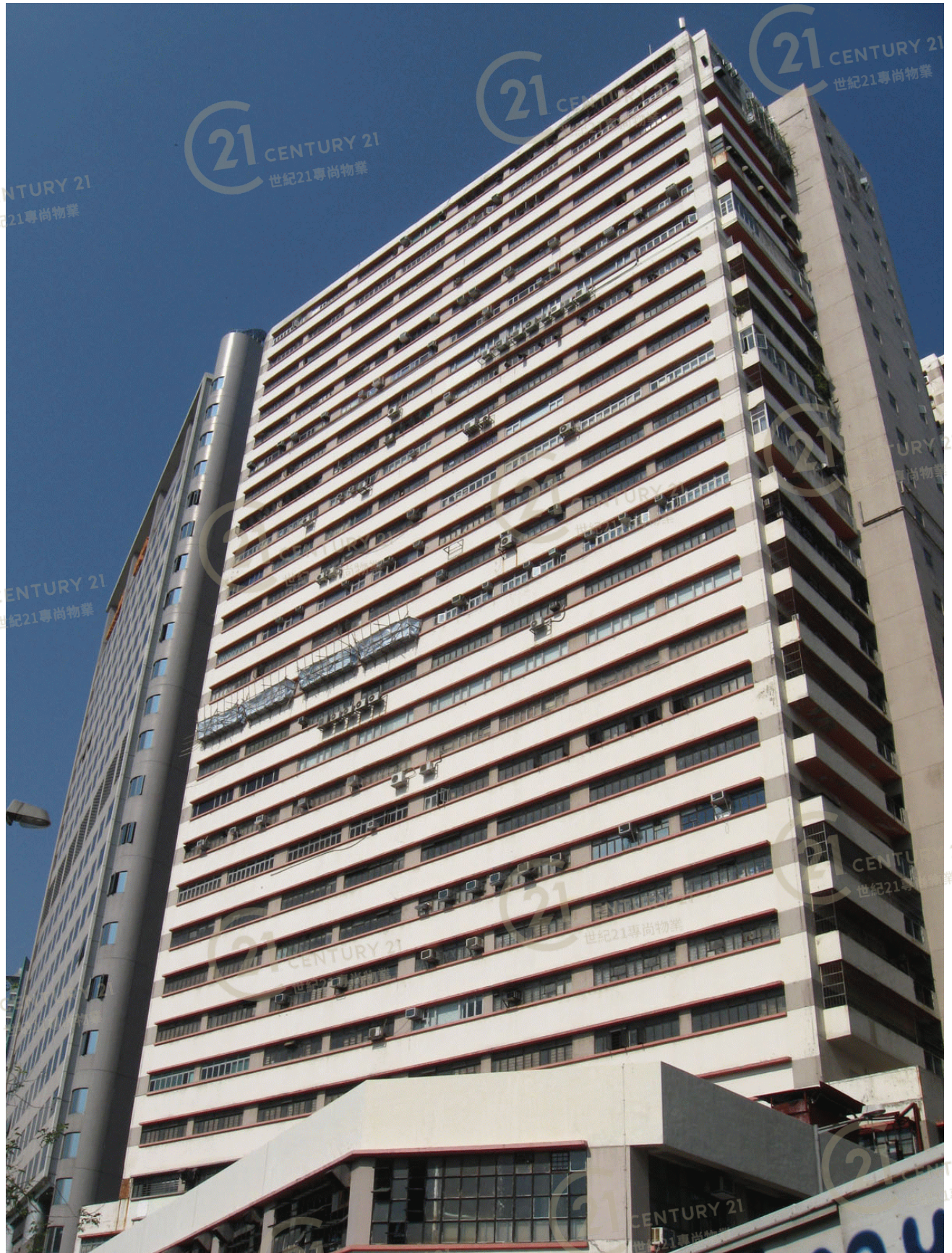
金發工業大廈1期 Kingsford Industrial Building Phase 1
