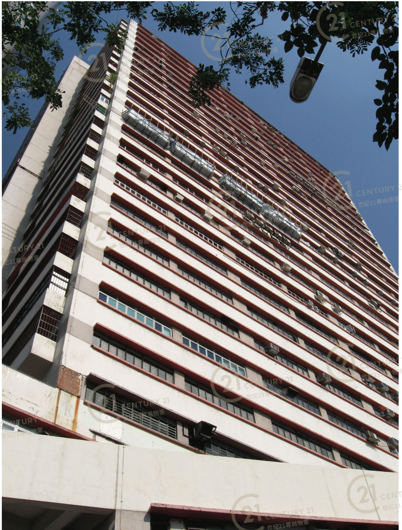
金發工業大廈1期 Kingsford Industrial Building Phase 1
