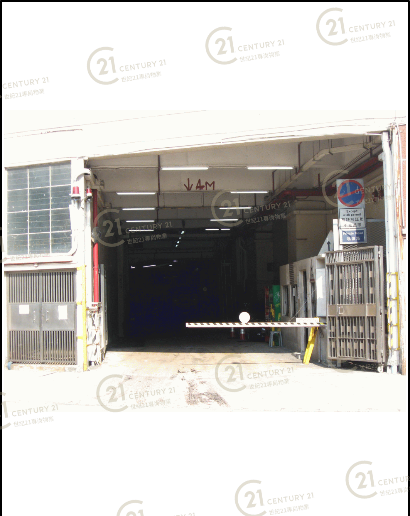
金發工業大廈1期 Kingsford Industrial Building Phase 1
