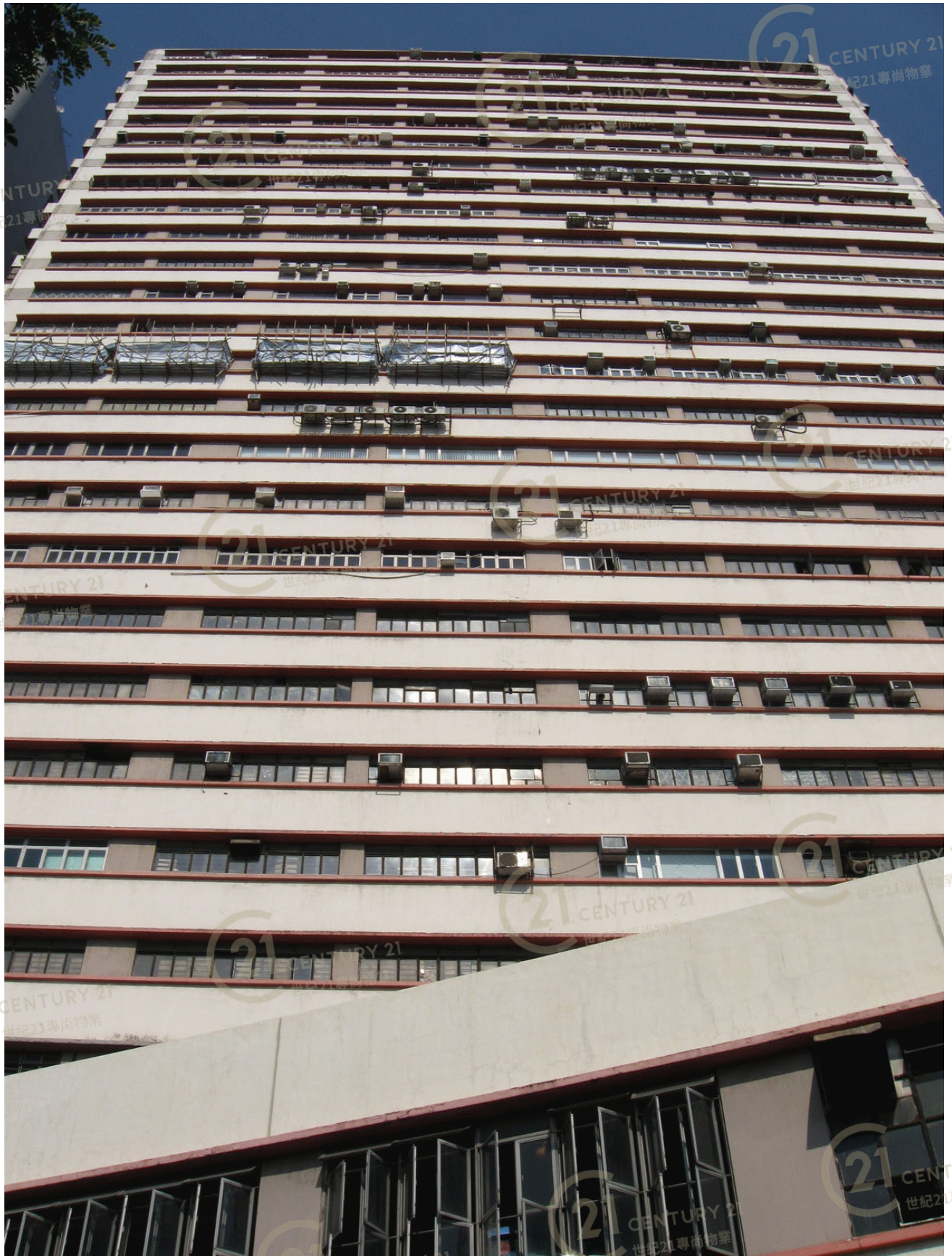
金發工業大廈1期 Kingsford Industrial Building Phase 1
