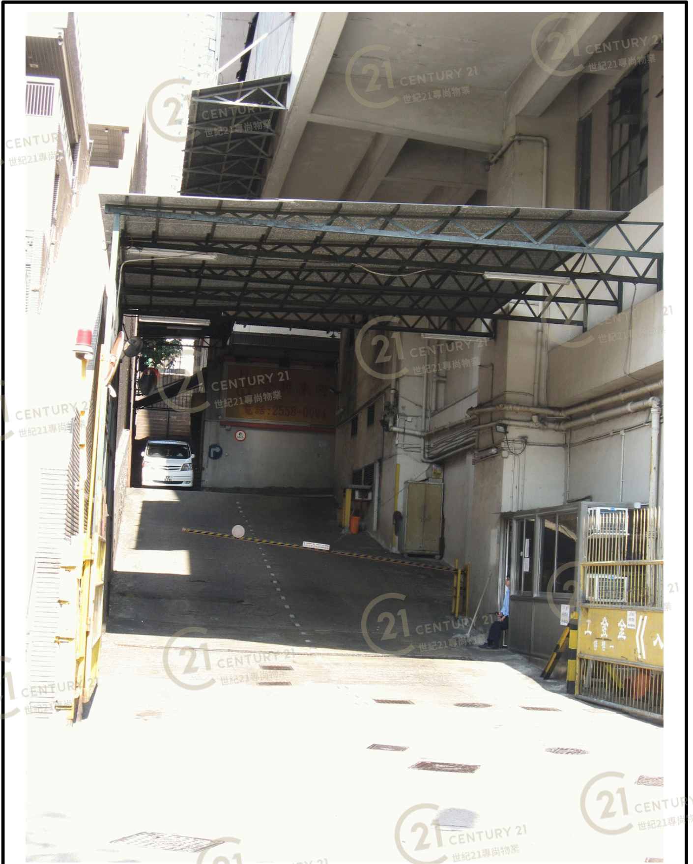
金發工業大廈1期 Kingsford Industrial Building Phase 1
