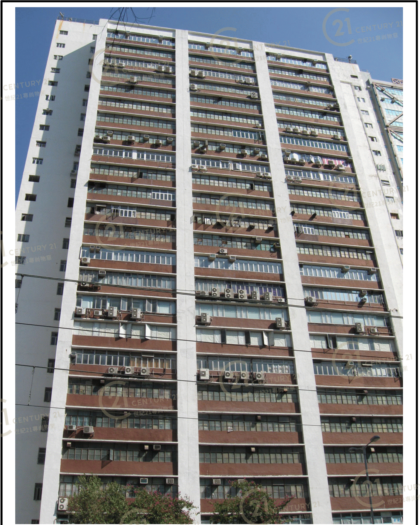
怡成工業大廈 Success Industrial Building
