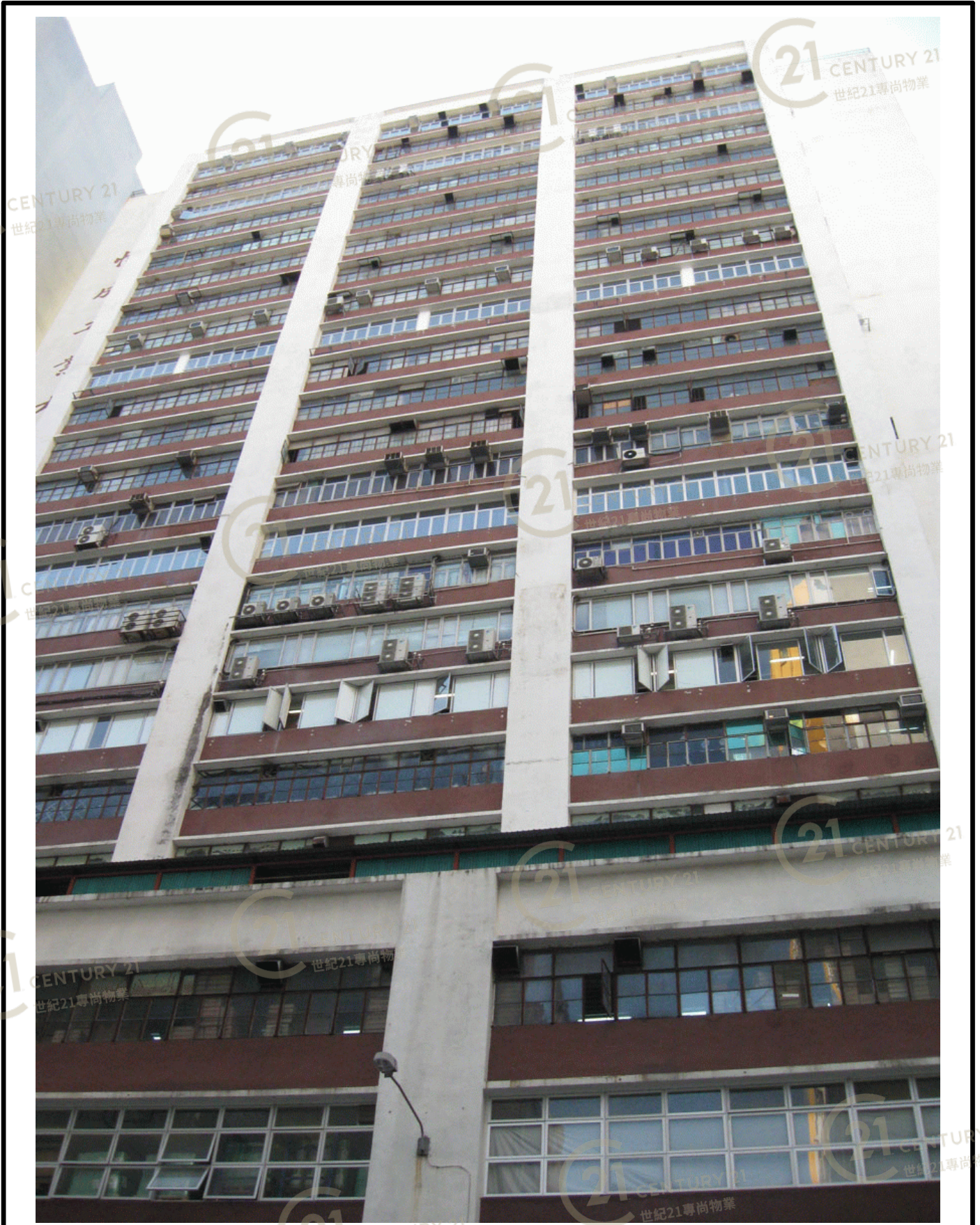
怡成工業大廈 Success Industrial Building
