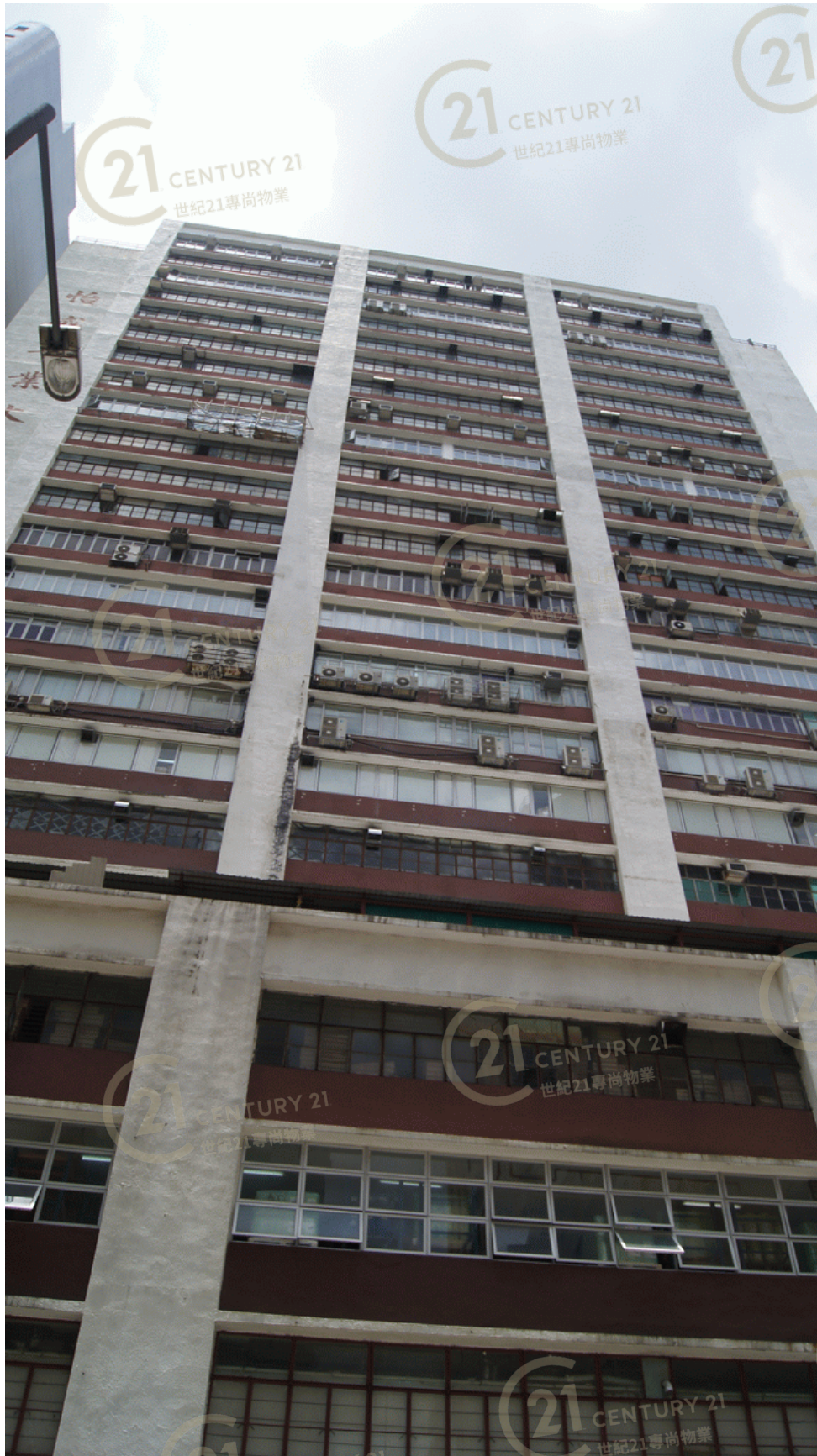
怡成工業大廈 Success Industrial Building
