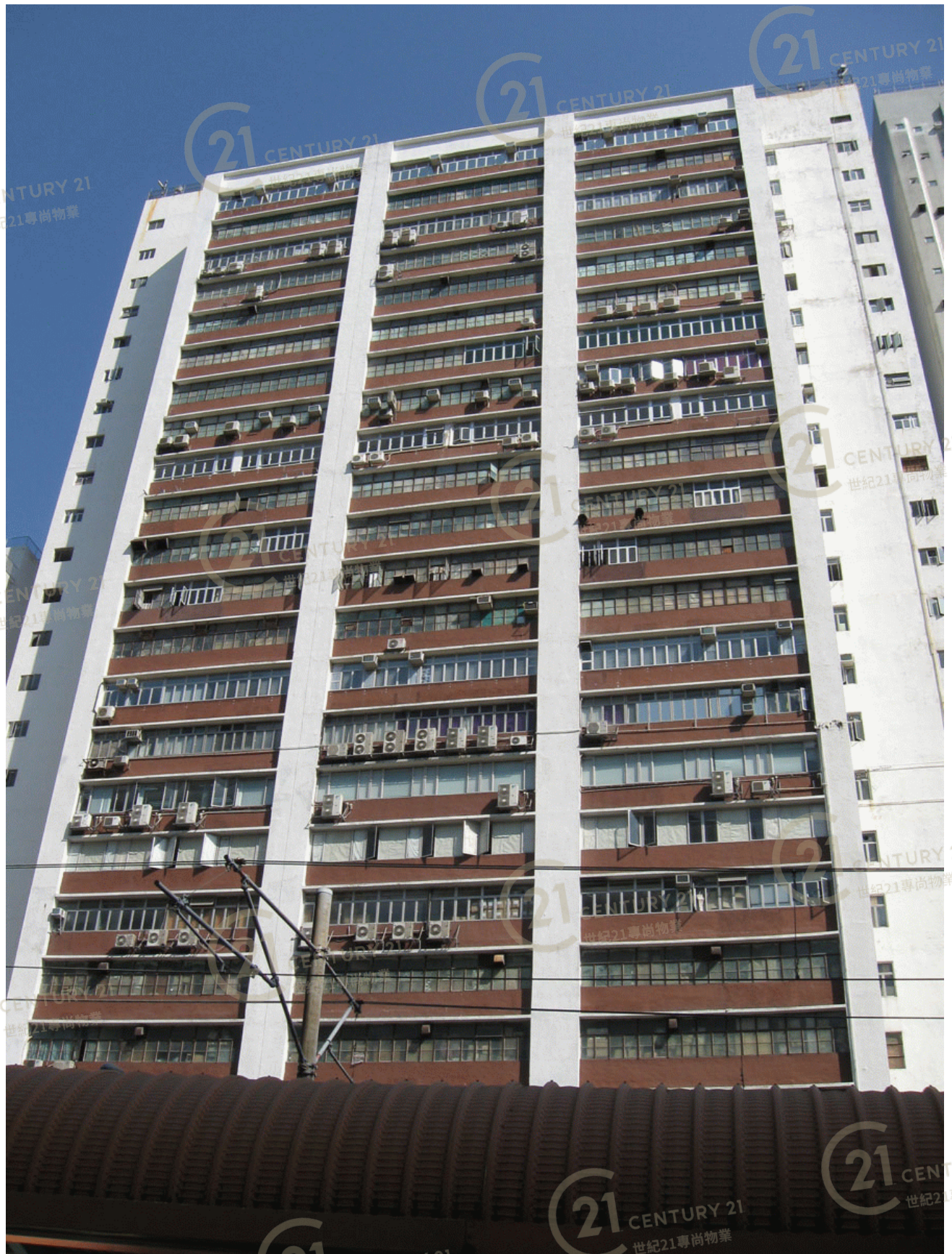
怡成工業大廈 Success Industrial Building
