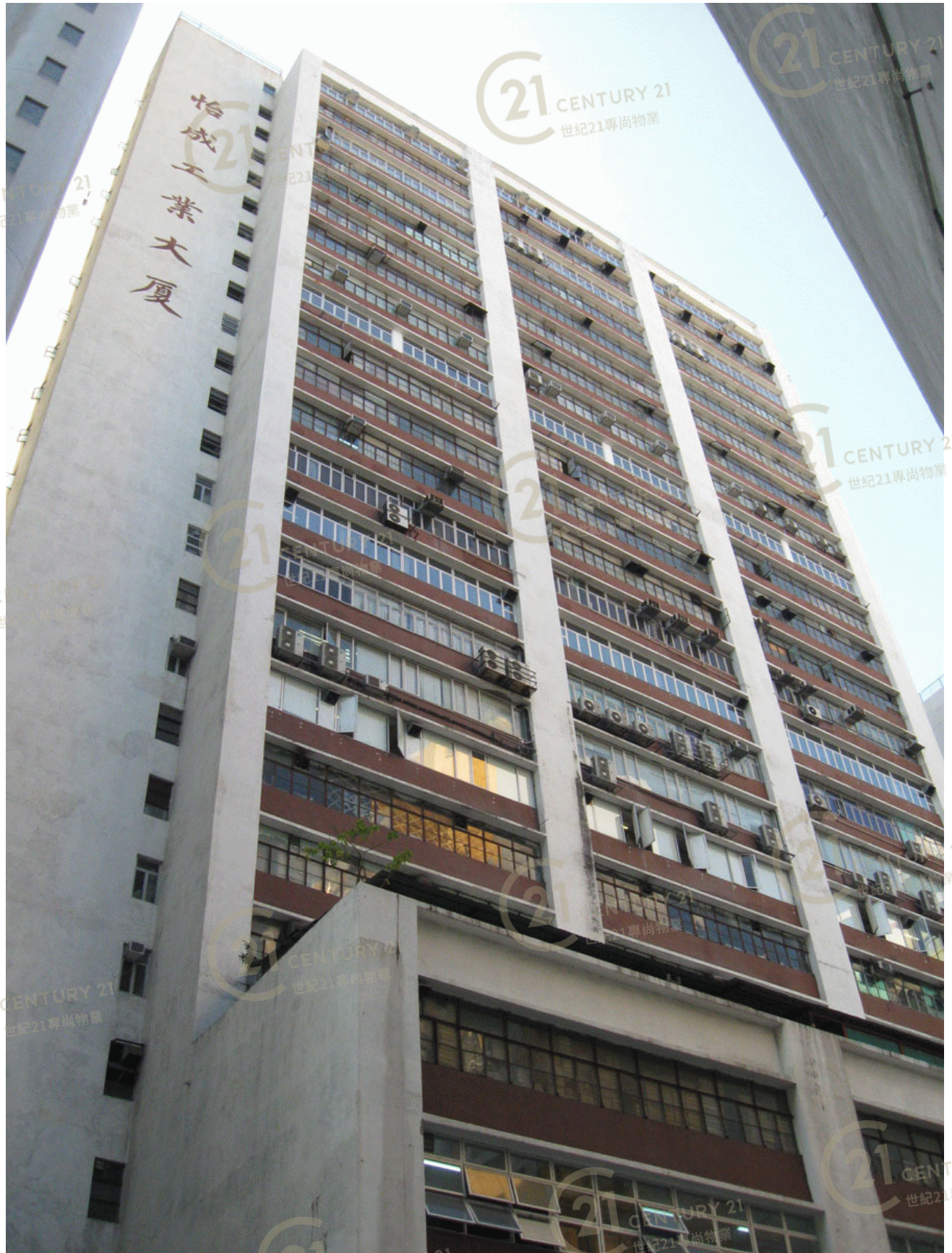
怡成工業大廈 Success Industrial Building
