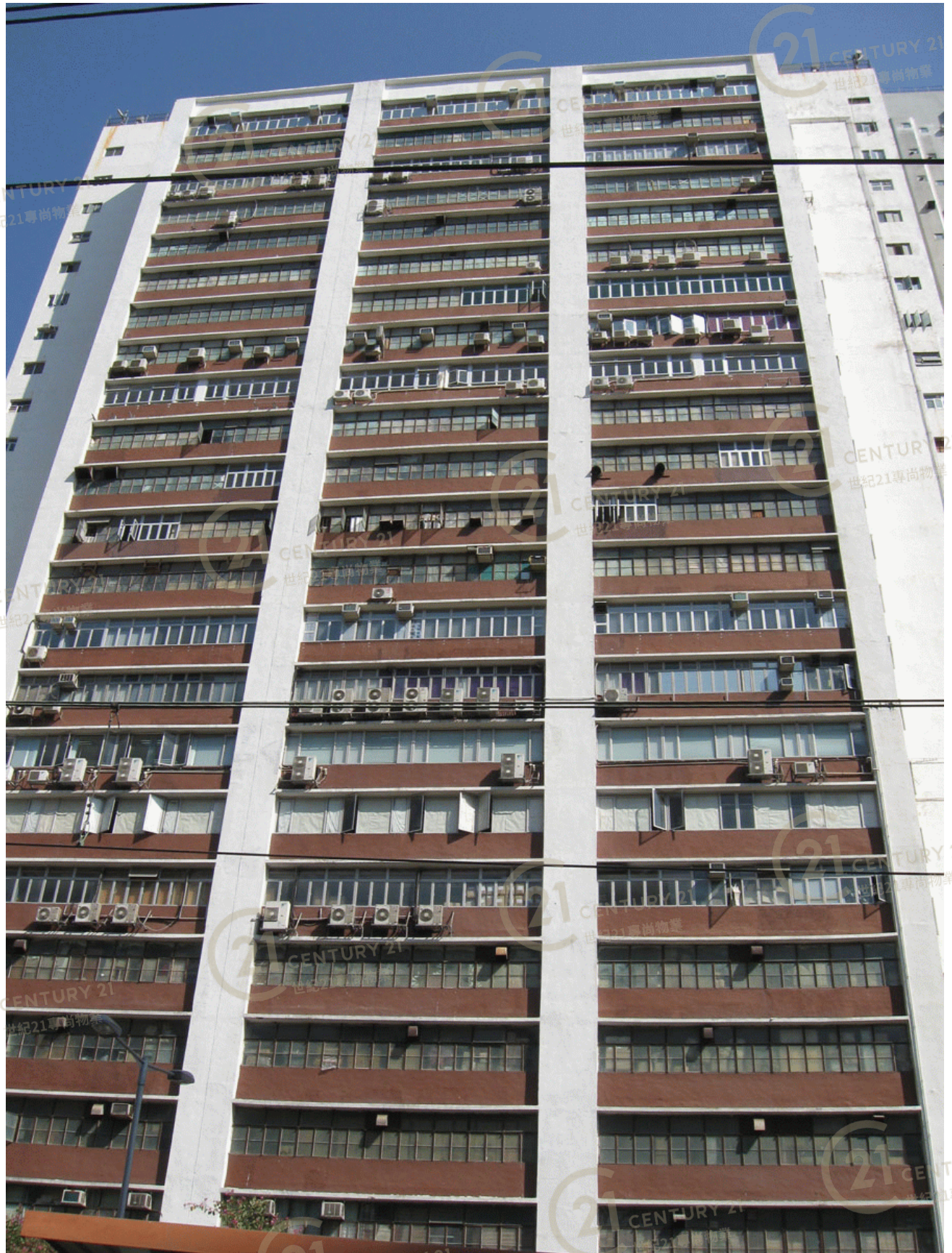
怡成工業大廈 Success Industrial Building
