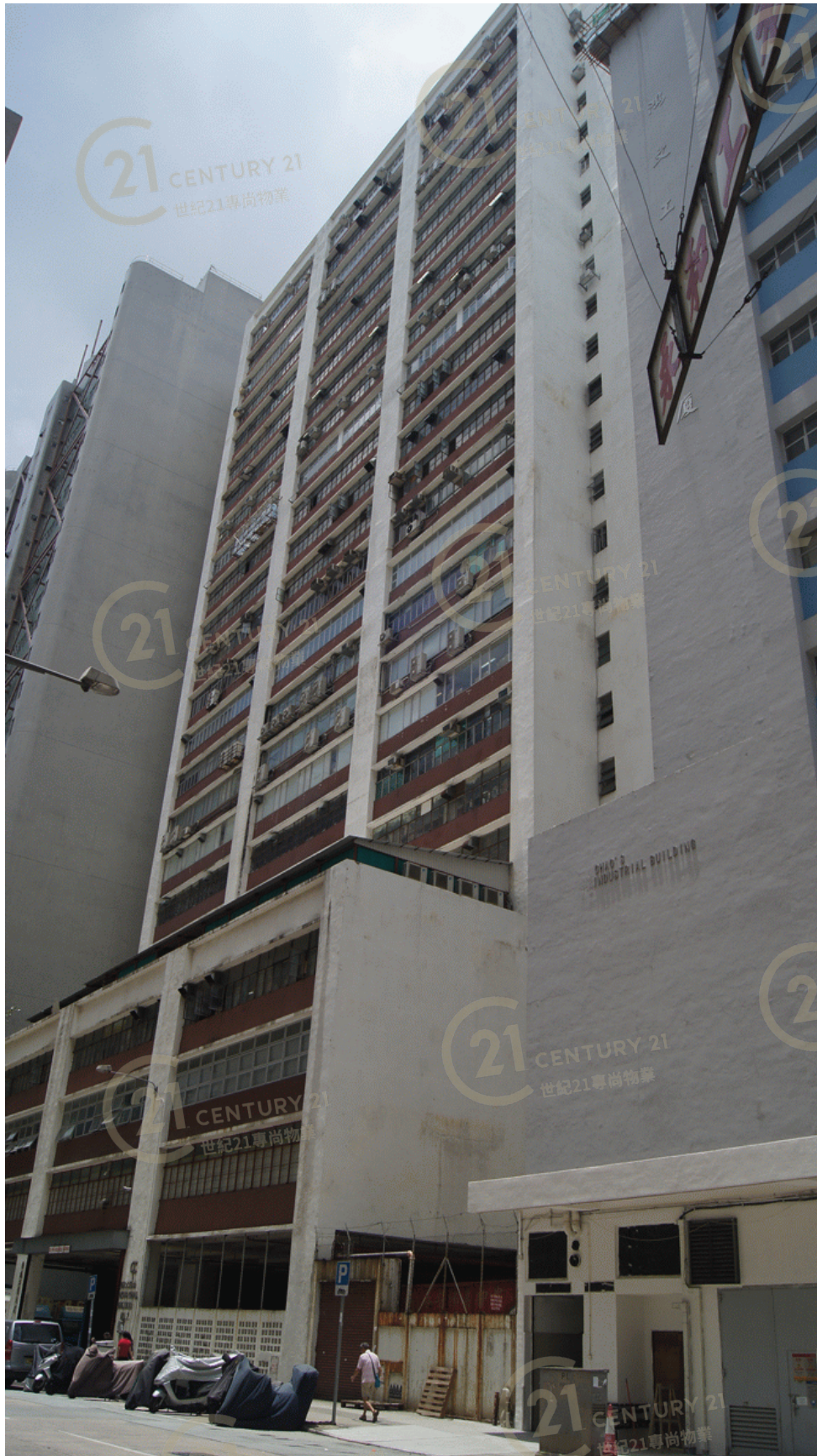
怡成工業大廈 Success Industrial Building
