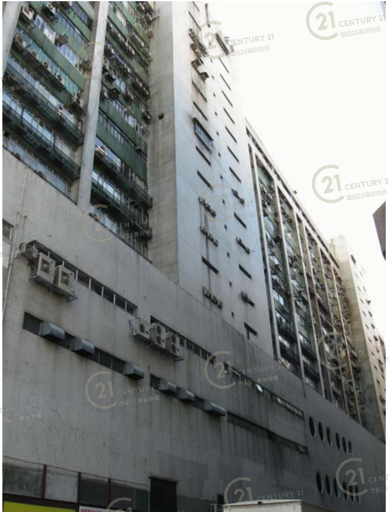
盈業大廈 Profit Industrial Building
