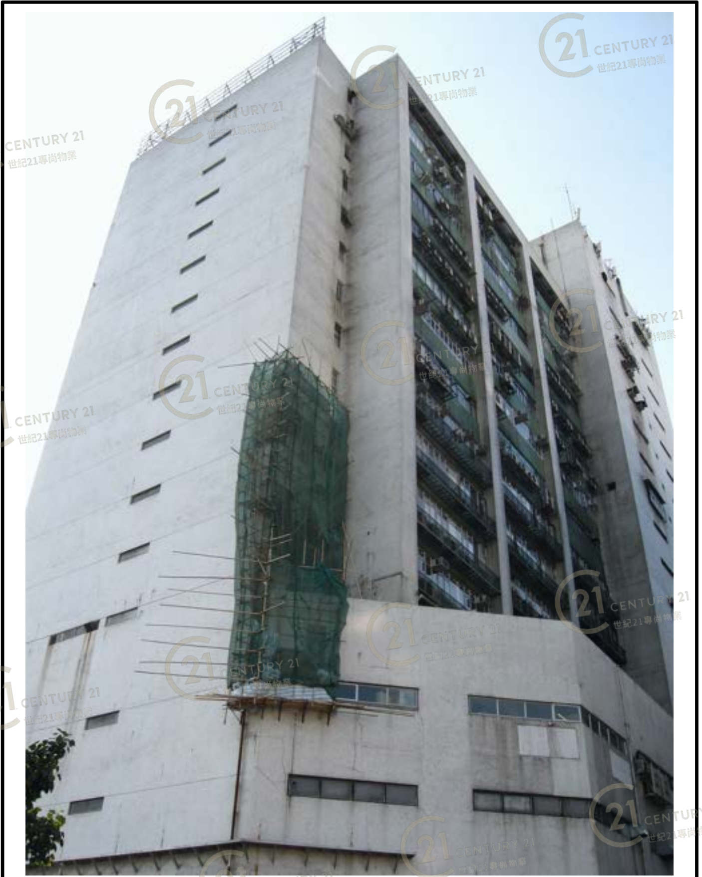
盈業大廈 Profit Industrial Building
