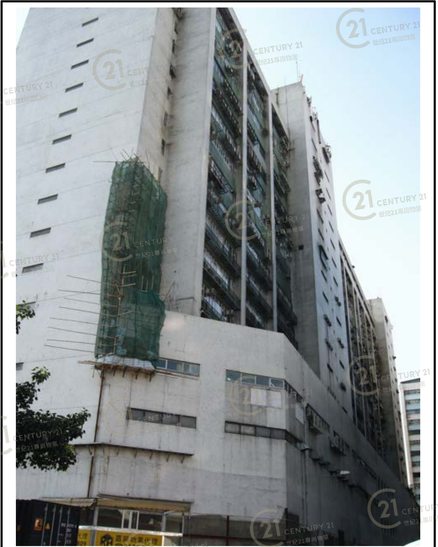
盈業大廈 Profit Industrial Building
