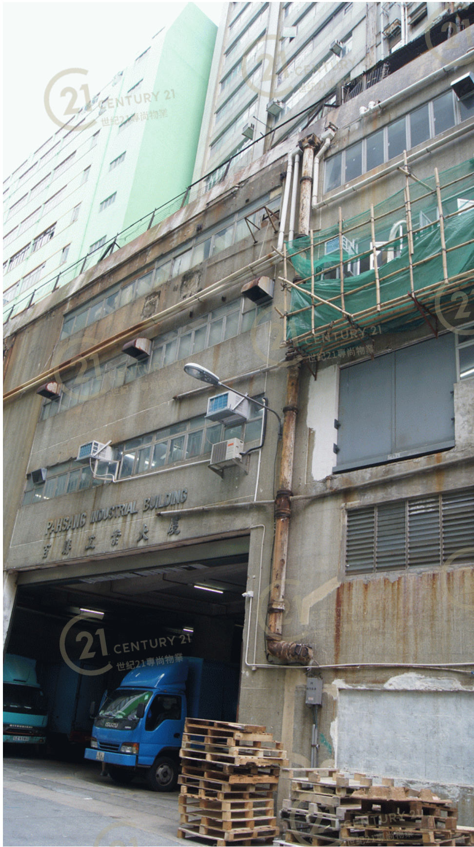
百勝工業大廈 Pahsang Industrial Building
