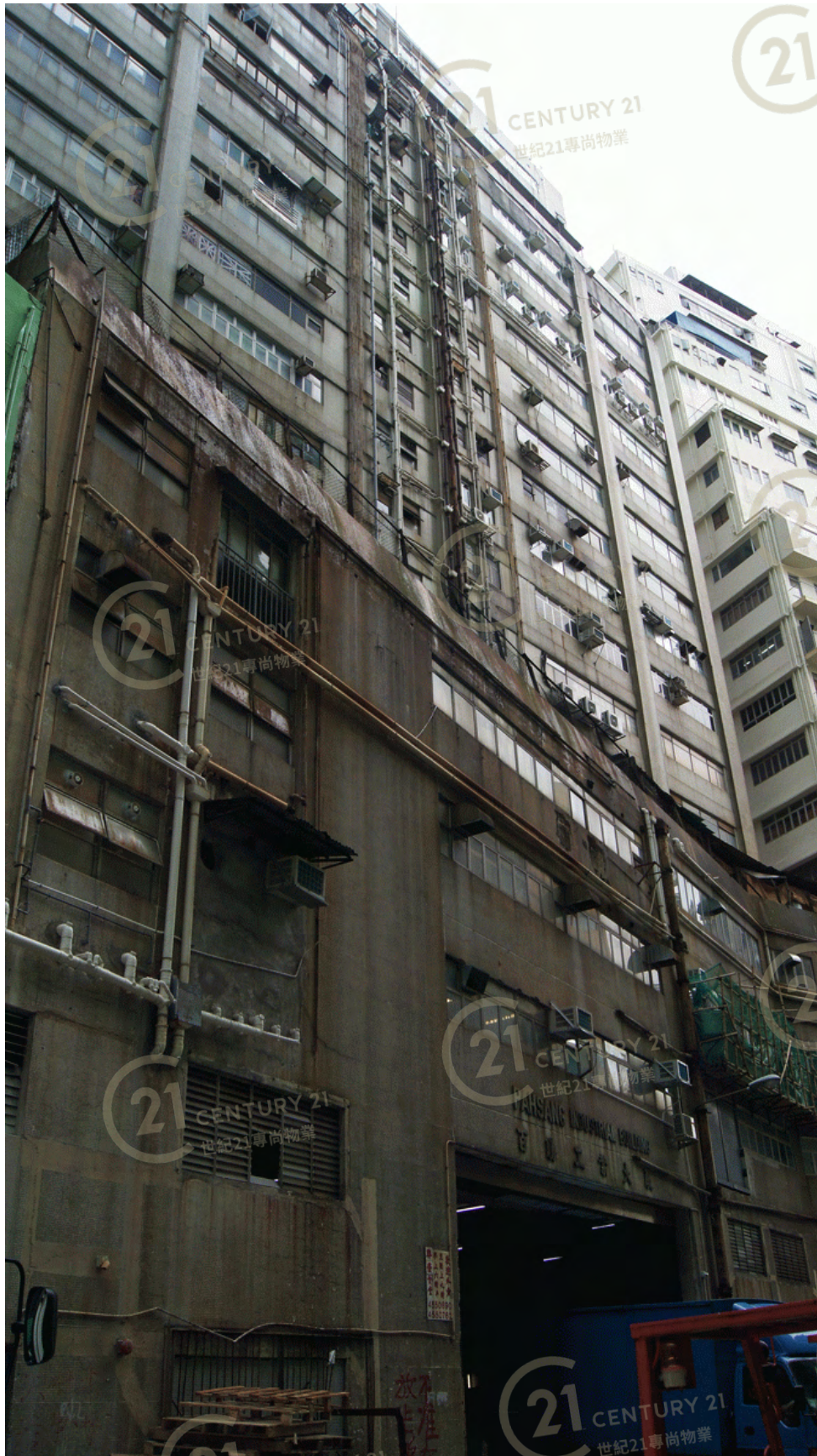
百勝工業大廈 Pahsang Industrial Building
