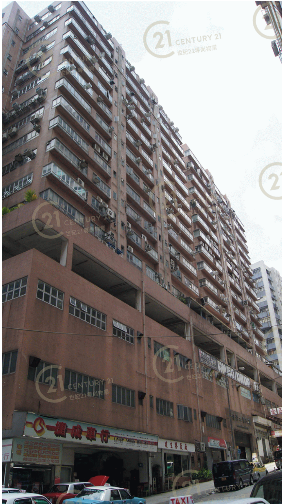
好景工業大廈 Goodview Industrial Building
