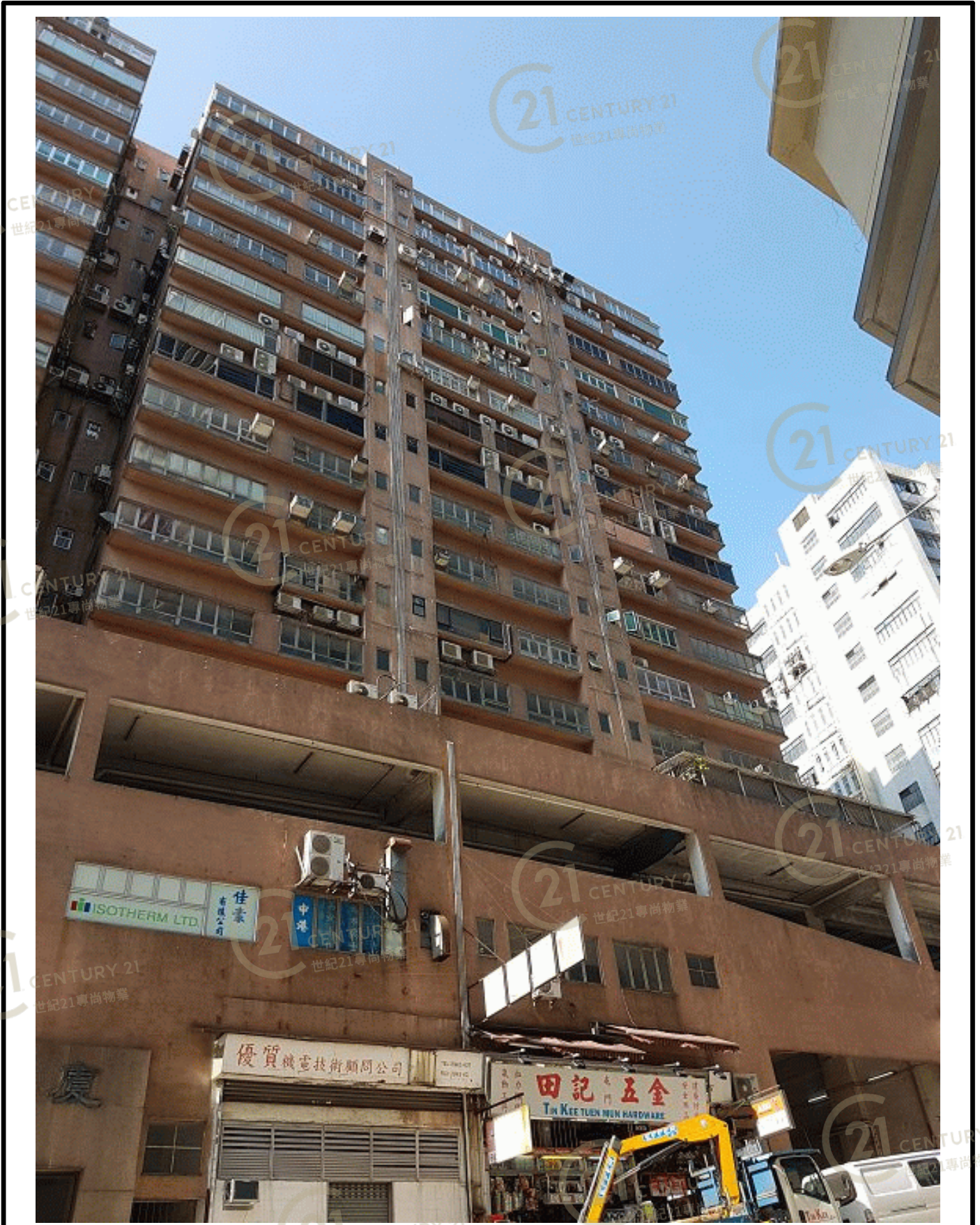
好景工業大廈 Goodview Industrial Building
