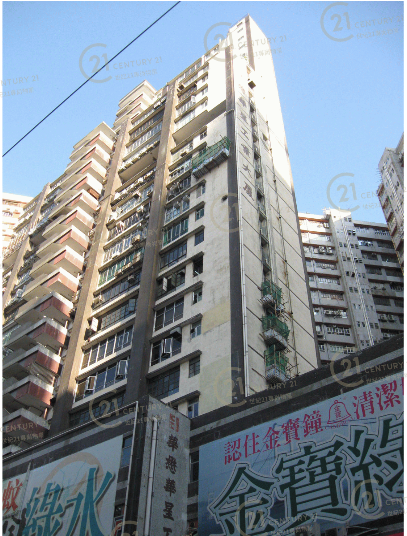
華星工業大廈 Wah Sing Industrial Building
