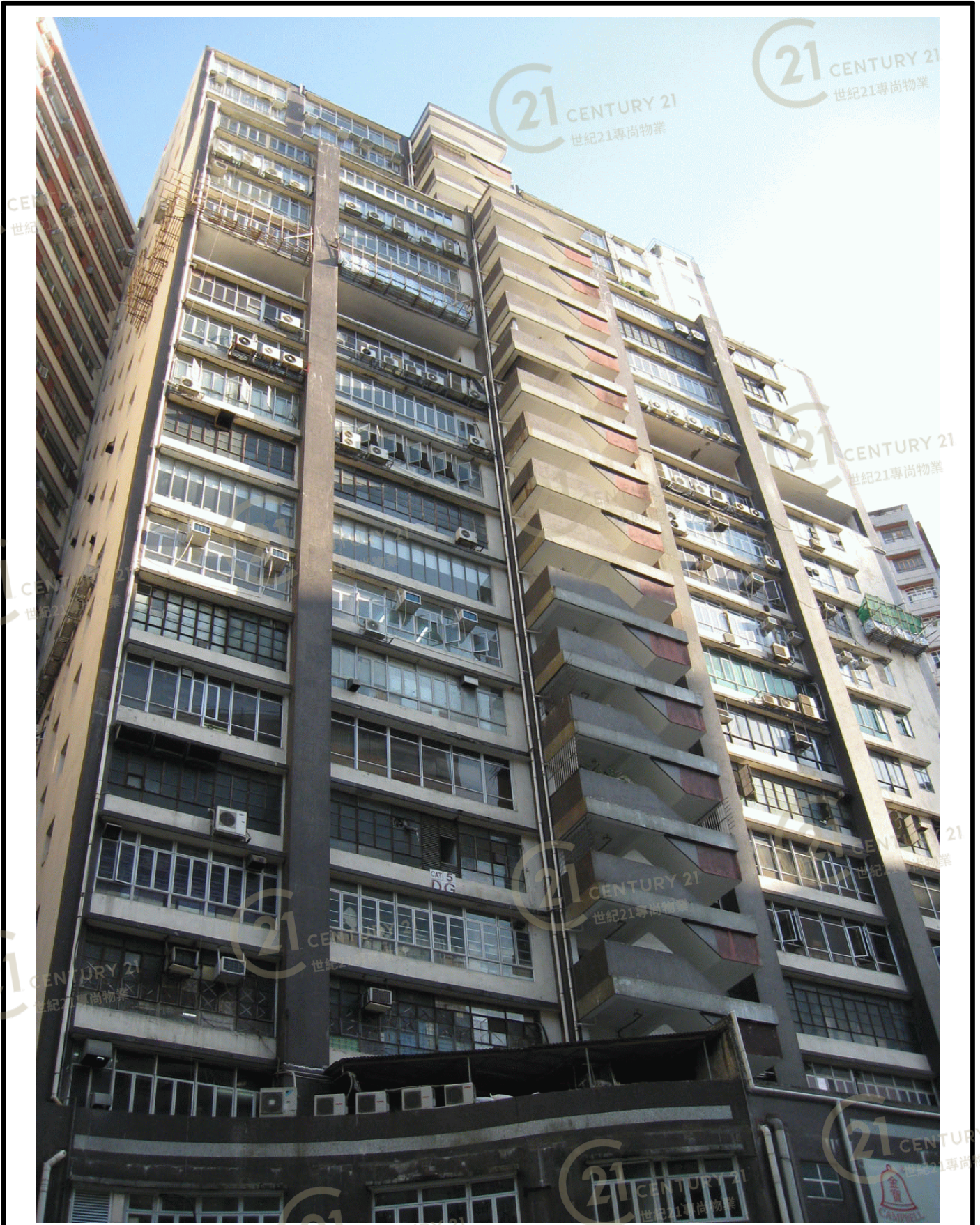
華星工業大廈 Wah Sing Industrial Building
