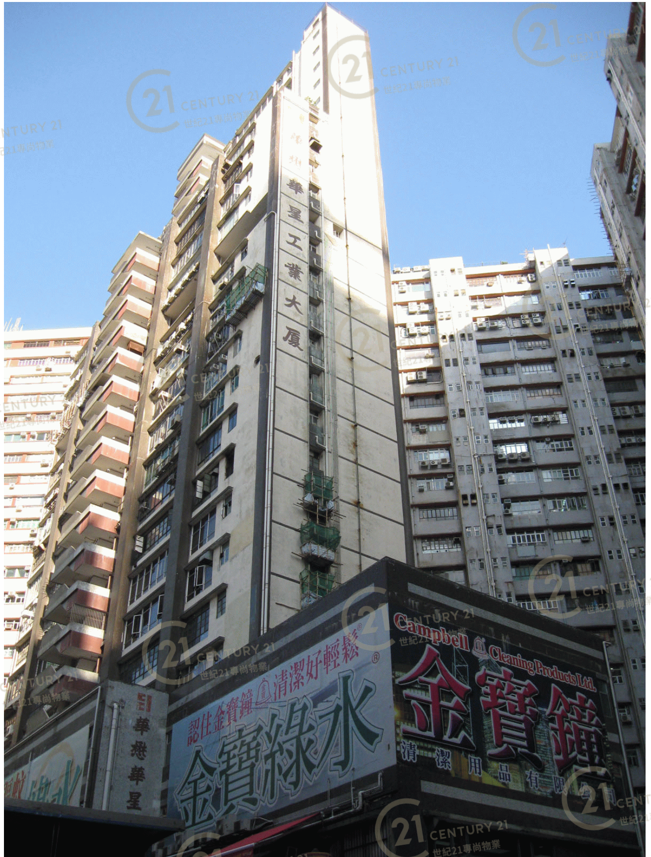
華星工業大廈 Wah Sing Industrial Building
