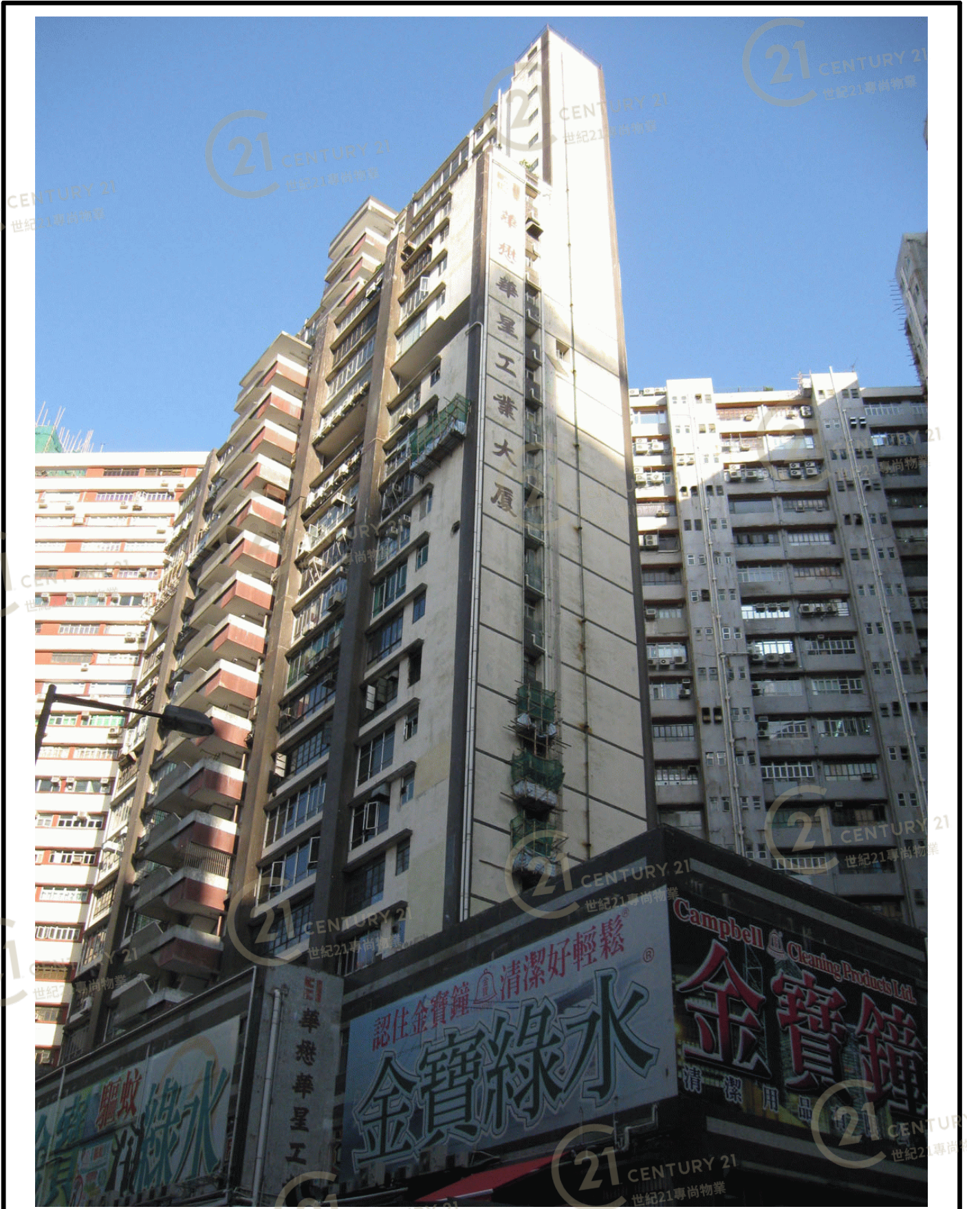
華星工業大廈 Wah Sing Industrial Building
