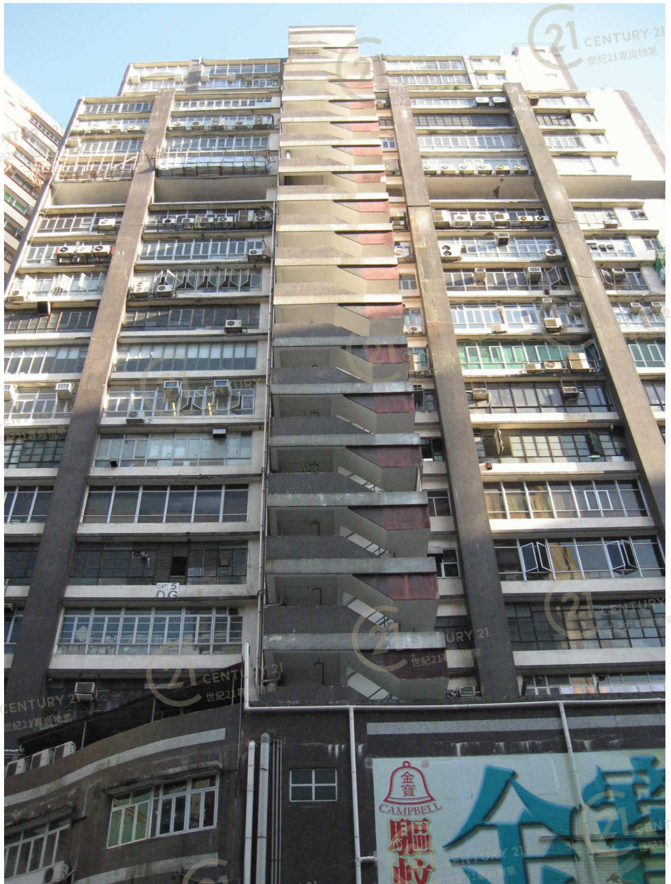
華星工業大廈 Wah Sing Industrial Building
